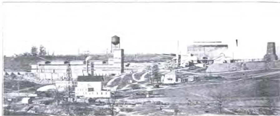
Ore Bin and Crusher Building
