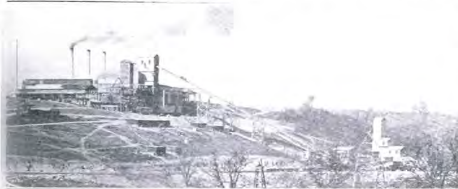
Power House Distillation Furnaces
