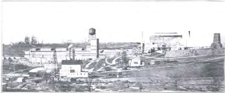
Ore Bin and Crusher Building
