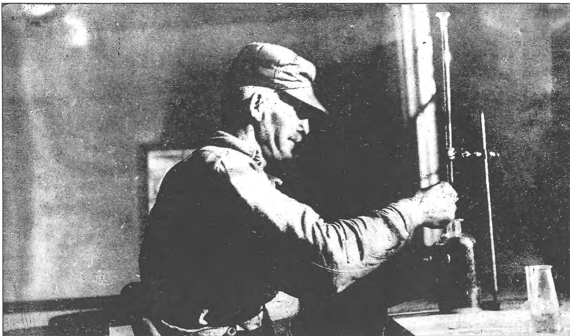
William Dearolph in the pump station of McDonald Dam Bavington, PA
