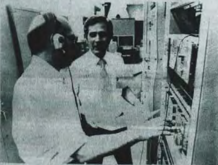
Testing the new T-1 carrier equipment here are Deane L. Bertrand, left, switchman for the Burgettstown office, and William
