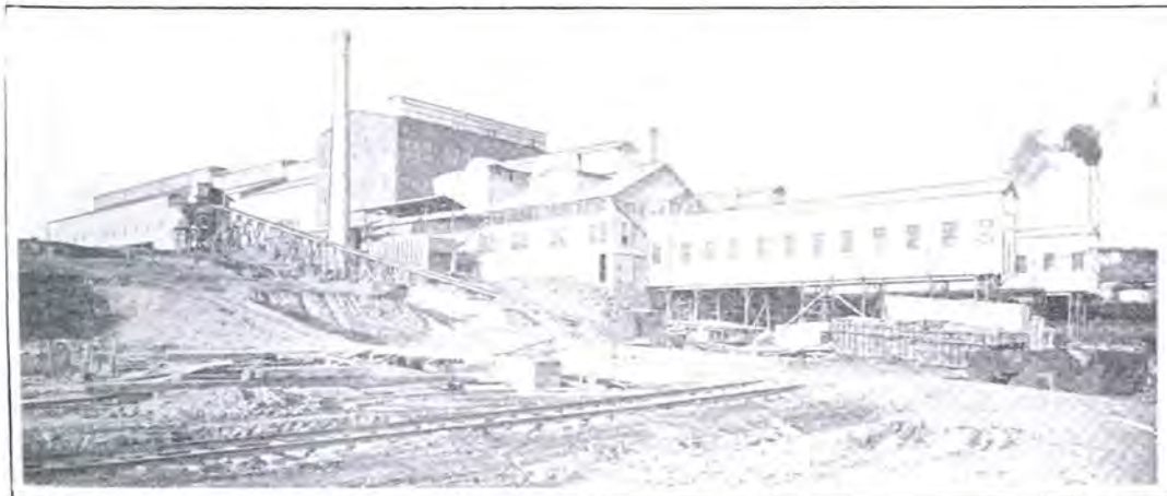
The Upper Picture Shows the Concrete Ore Bins and Ore Crusher Building. In the Lower Are Shown the Roasting Furnaces with the Chamber Acid Plant to the Left
