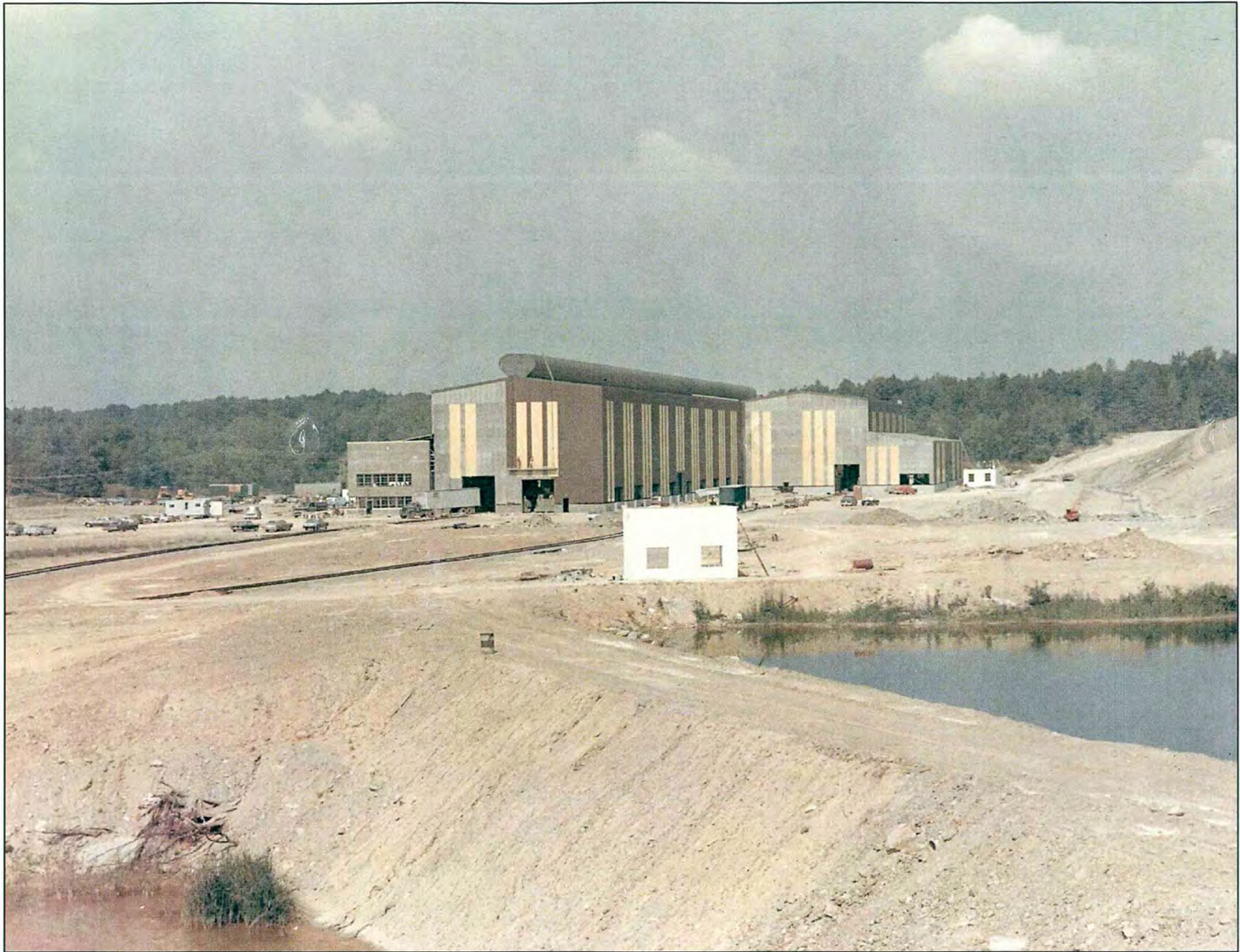
Union Electric Steel, Harmon Creek Industrial Park Photo taken from haul road near the truck garage looking west.
