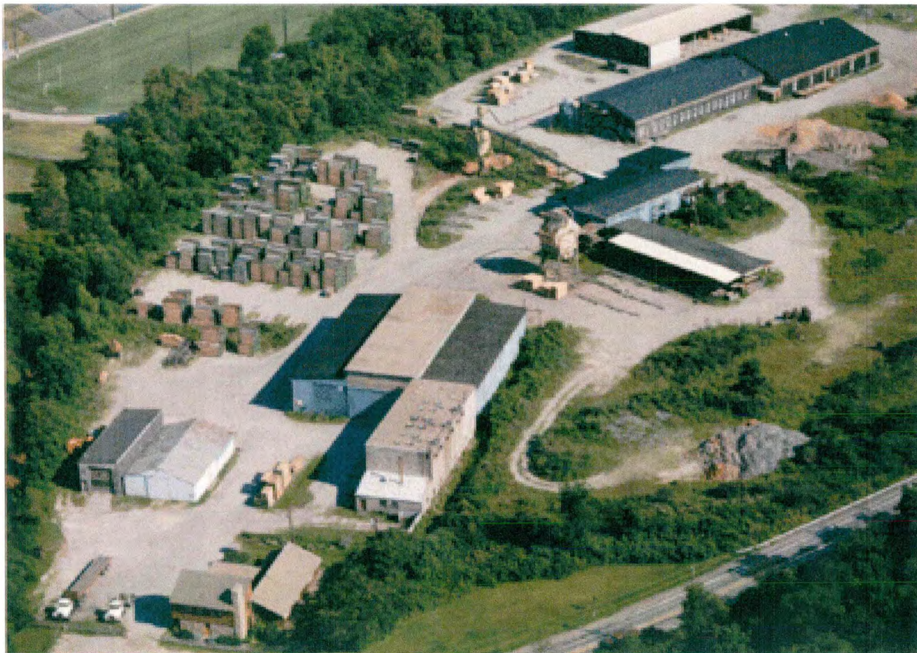
Ariel View of Sutherland Lumber Burgettstown, PA
