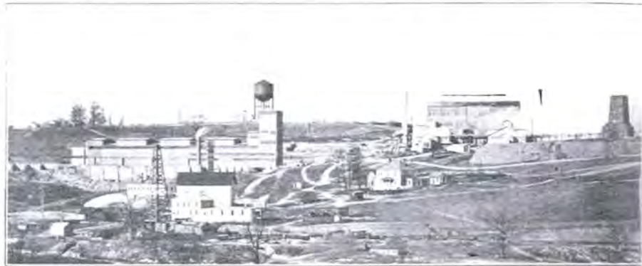
Ore Bin and Crusher Building
