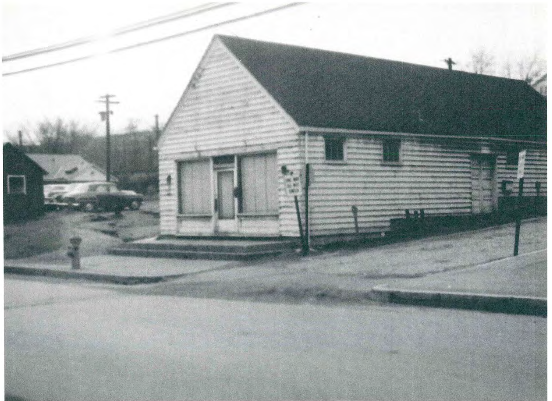
Yukevich Building was razed to Build Gulf Service Station-Main Street Location was between the Burgettstown Post Office and the Bank.
