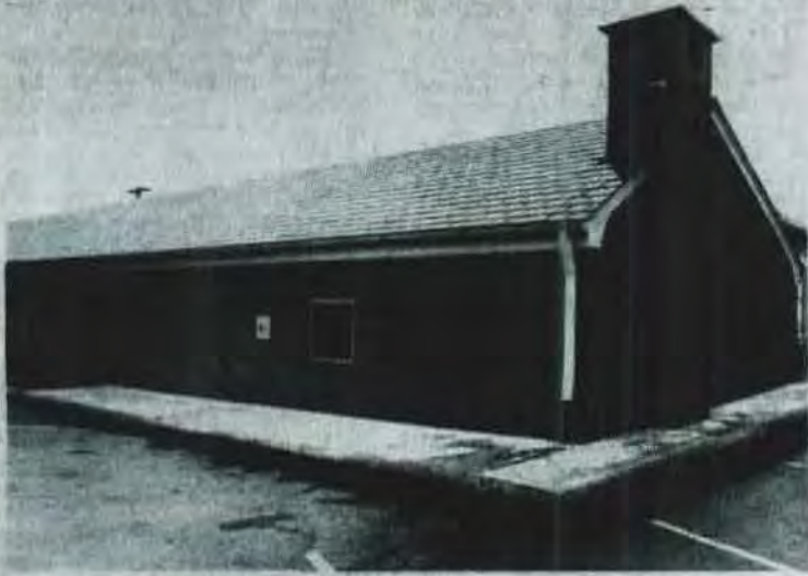
This will be the new and completed installation here.
