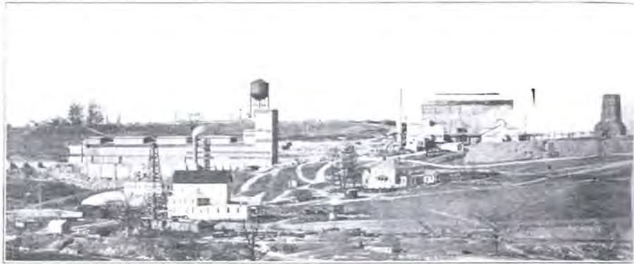
Ore Bin and Crusher Building
