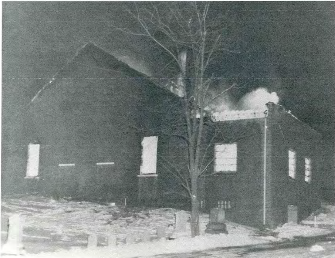
Florence Church Destroyed by Fire-February 1963
