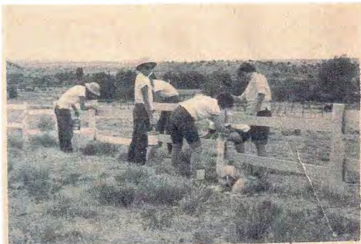
This photo shows the group at work painting the fence around the Navaho cemetery. Previous to the painting project, they had rebuilt and repaired the fence. Because of the existing Navaho superstitions concerning death and burial, they refuse to enter the cemetery, much less maintain it. The nearby Mission is informed of any death among the Indians, and it is left in the hands of the Missionaries to bury the remains. The group here is giving the fence
