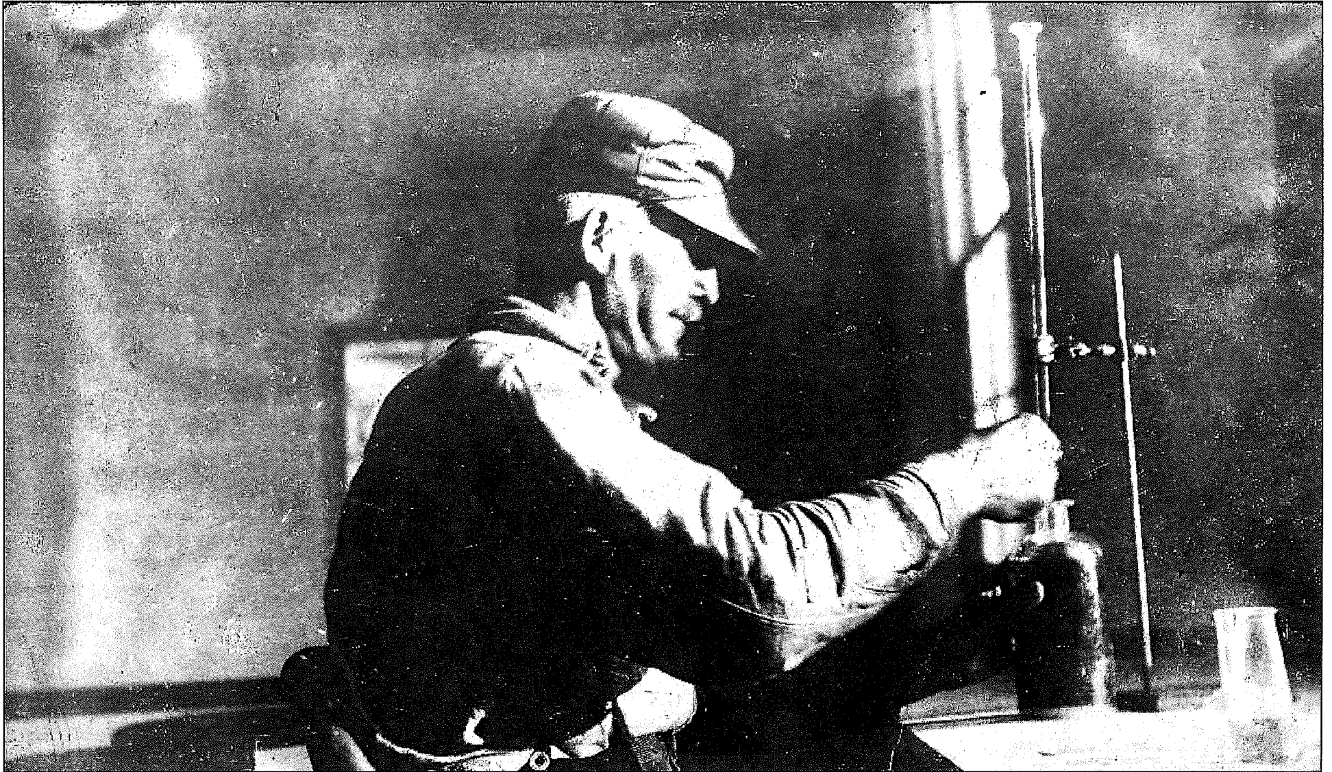
William Dearolph in the pump station of McDonald Dam Bavinton, PA
