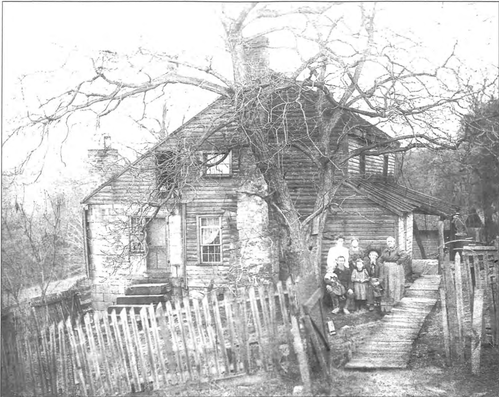
Evan D. Hindman Homestead Hall's Road, Brooke County, WV
