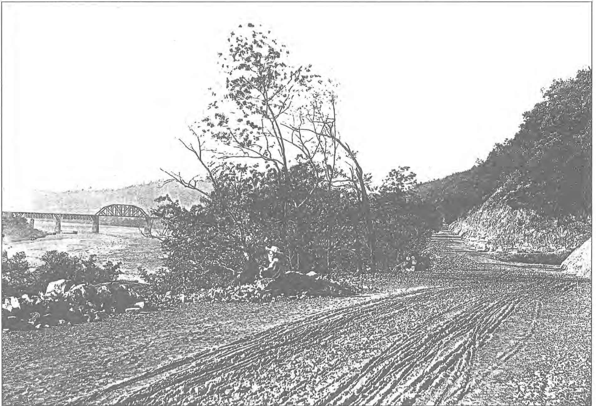
Preparation for the street car lines to connect the future WV Rt. 2 to Steubenville, Ohio.
