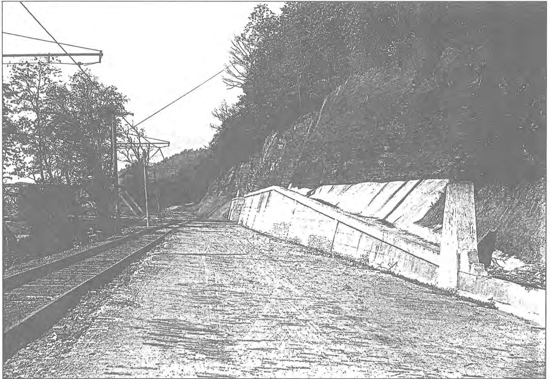
View approaching the street car tracks near Steubenville Bridge from Follansbee, WV. -Abt. 1904
