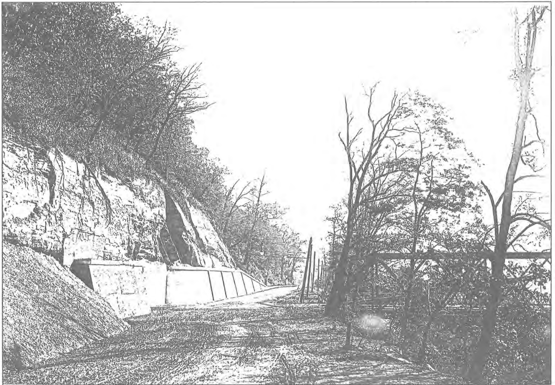
The entrance of Steubenville Bridge on right, connecting WV Rt. 22 and the Steubenville-Abt. 1904.
