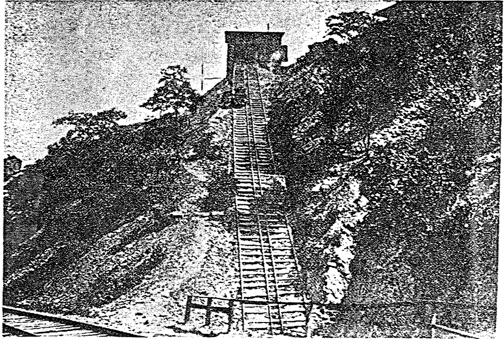
Incline leading to clay mines
