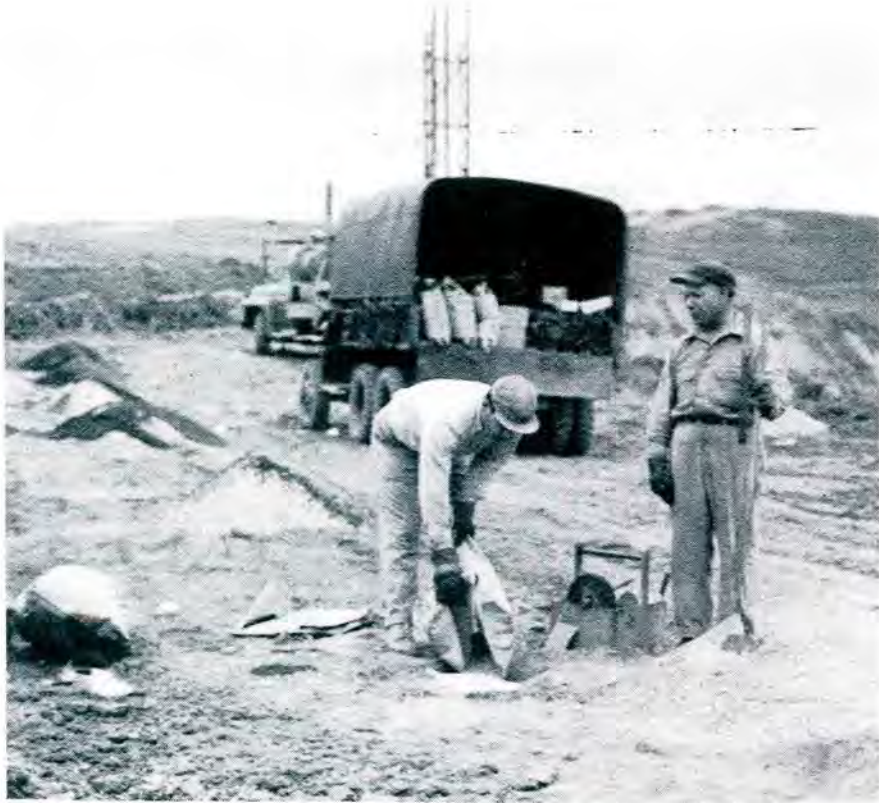
Holes are charged with ammonium nitrate mixed with fuel oil. Supplies are carried in truck in background.
