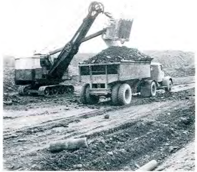
Raw coal stockpiled adjacent to the haulage road is reloaded into 22-ton tractor-trailer units by this 2-cu-yd shovel.
