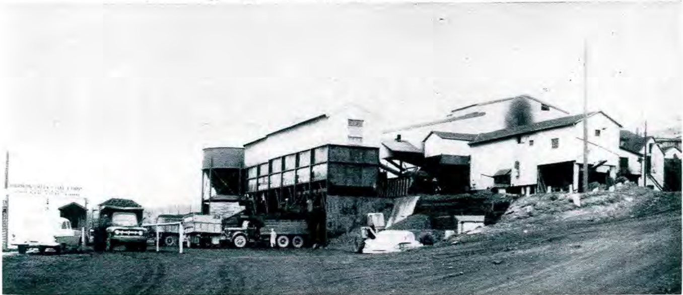
View of truck-loading section, which handles more than one-half of annual plant output.
