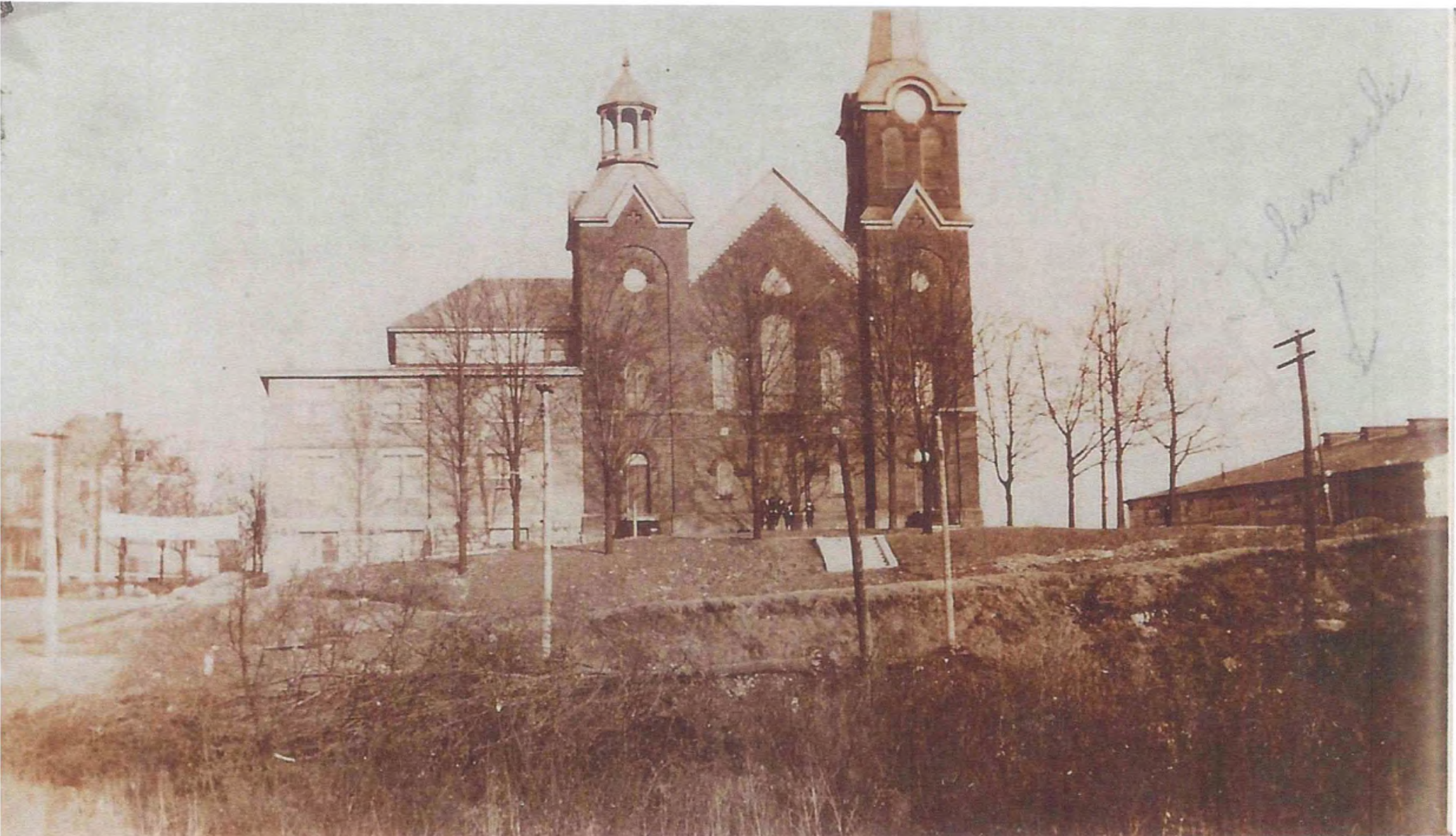
Hillcrest Presbyterian Church-after addition Main Street, Burgettstown, PA
