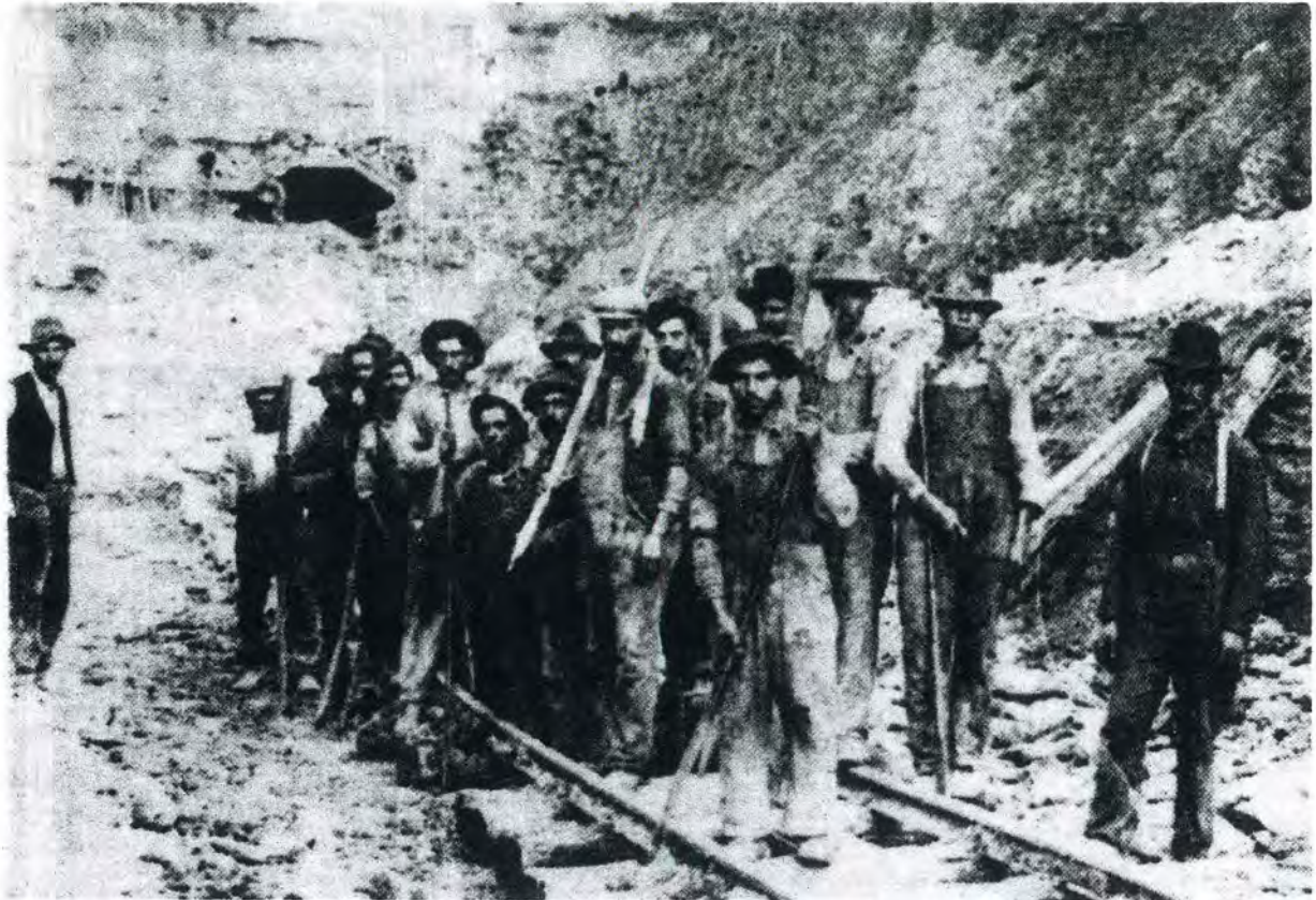
A group of workmen pause to face the camera of Frank France of West Middletown in 1903, during construction of the Pittsburgh and West Virginia (Wabash) Railroad.
