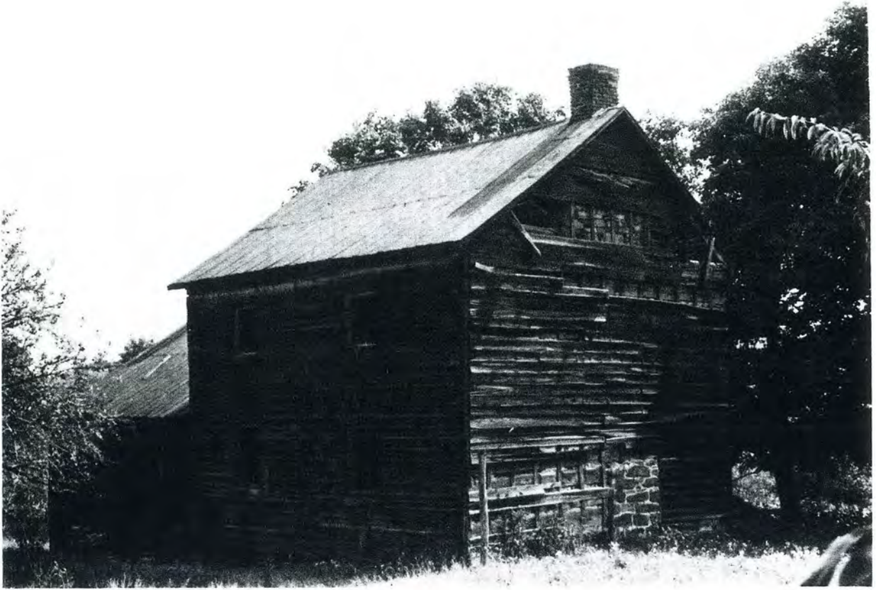
McCready Log House in Jefferson Township - Built in 1785. Removed to Meadowcroft Village - 1975.
