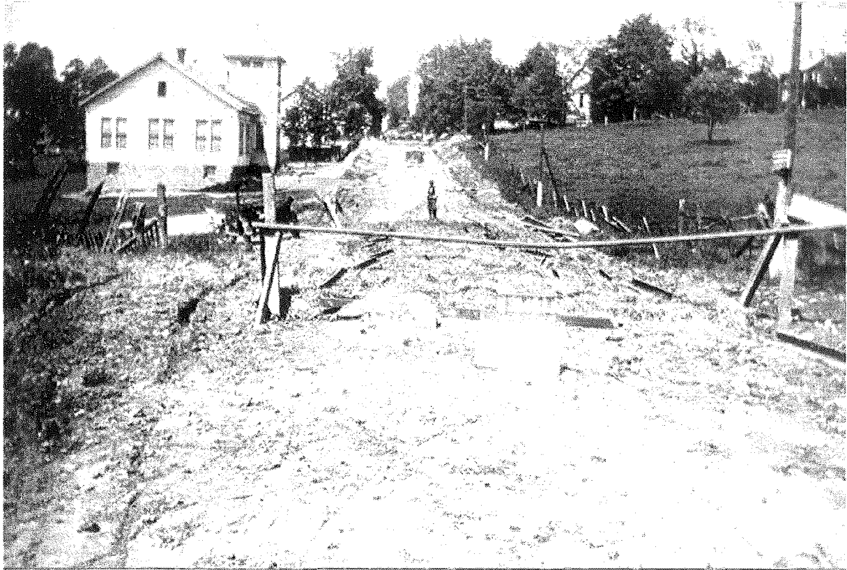
Construction of the Washington Pike through Independence Village
