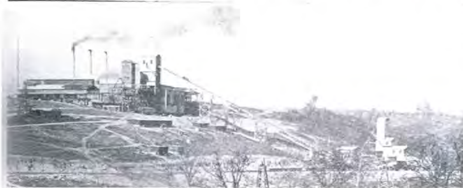
Power House Distillation Furnaces
