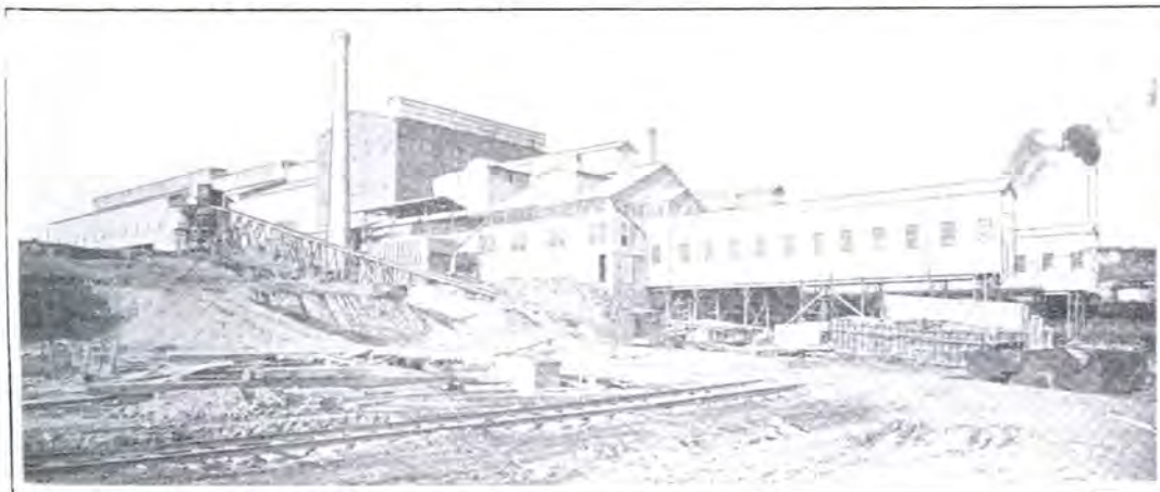
The Upper Picture Shows the Concrete Ore Bins and Ore Crusher Building. In the Lower Are Shown the Roasting Furnaces with the Chamber Acid Plant to the Left
