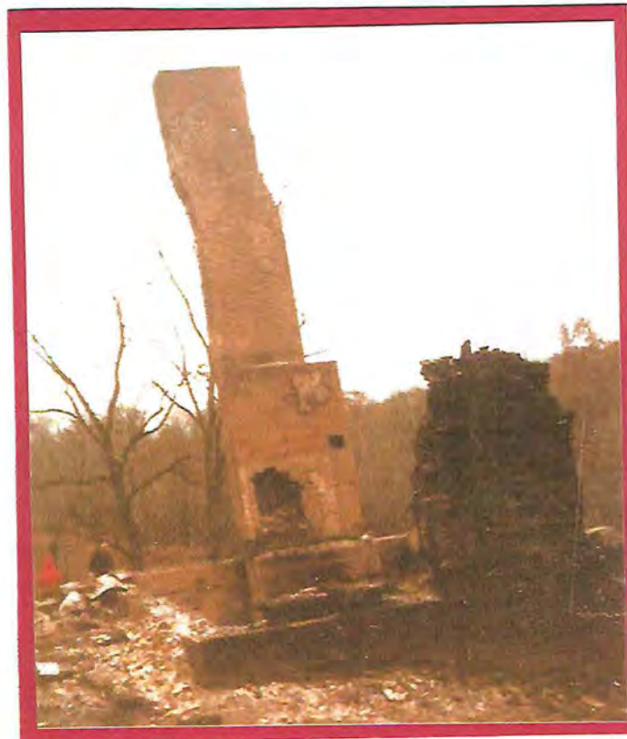
The crooked chimney left standing after the fire school burned the house.
