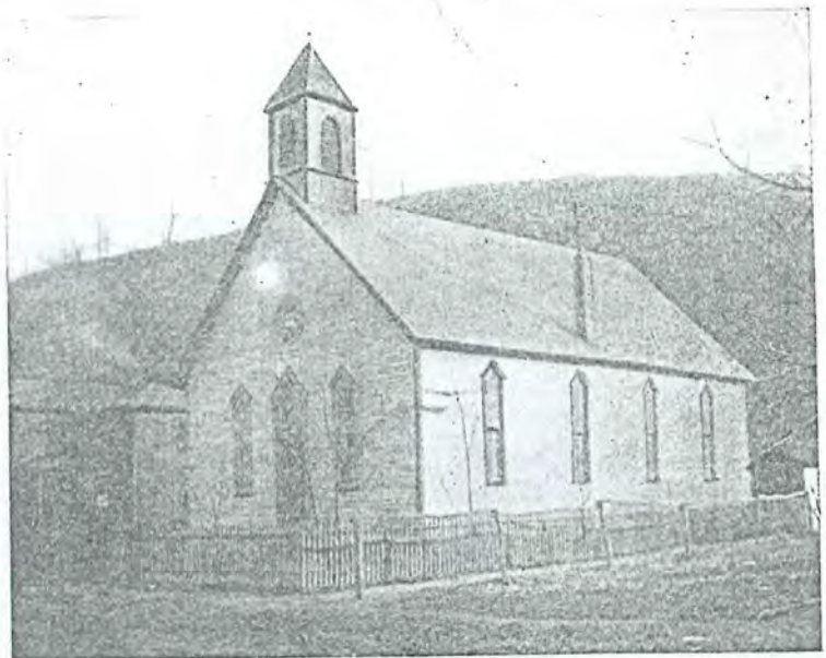
METHODIST CHURCH OF COLLIERS W. VA.
