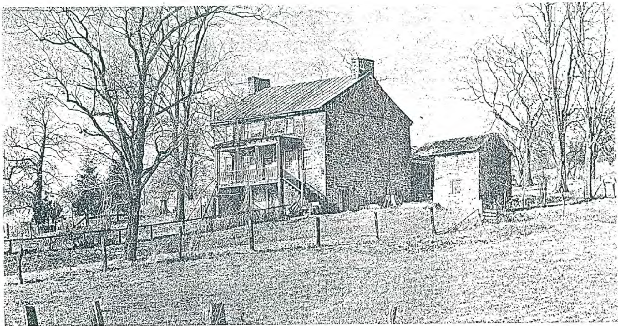
ODDITY. The Patterson home in Avella, Washington County, is little changed from its original appearance. Built in 1794 of rough-hewn native stone, the walls are almost two feet thick. "Oddity" was the name William Patterson gave to his odd-shaped parcel of 245 acres. His patent was signed by Benjamin Franklin.
