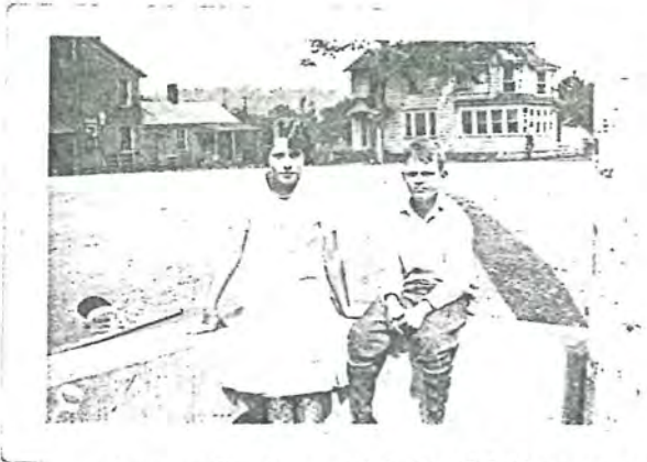
One of the old Todd houses
