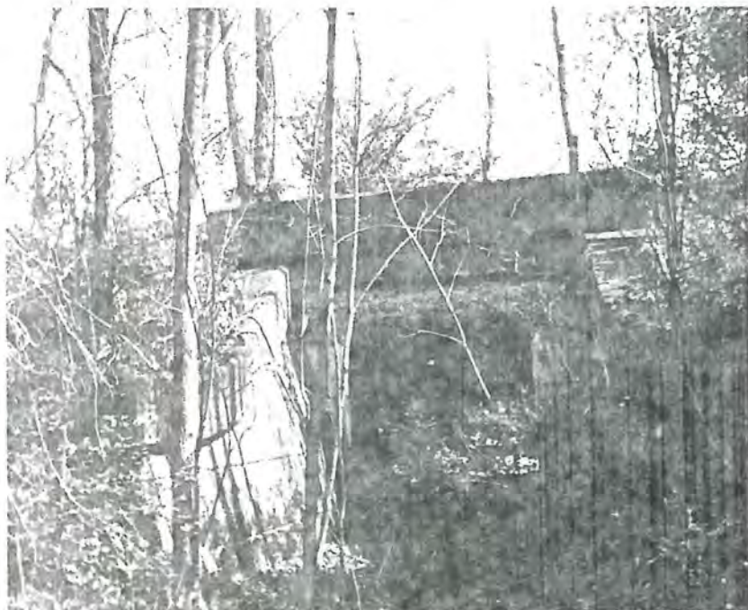
PASSENGER WALKWAY under tracks at Hanlin. Constructed circa 1910 following the tragedy of the Flem- ing family in 1904. The arch and the walkway are side by side, about 200 feet east of the steel bridge. During summer months, foliage and brush fully obscure it from view.
