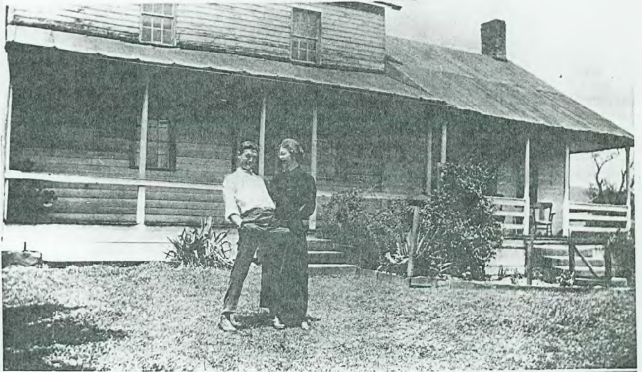
Robert McCready Homestead. Pictured are Lorin and Margretta Melvin McCready, the last of the McCready family to occupy it. The log part of the house was probably the first log house built in Jefferson Township. Pioneer Robert McCready was its builder. In his journal he states that he built it not far from the Mingo Trail.
