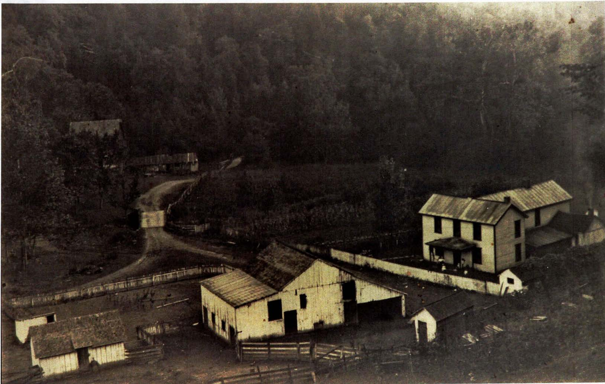
Panoramic view of Kidd's Mill. Mill in upper left of picture. Boarding House lower right. Picket fence washed put in 1912 flood. Stables and outbuildings in foreground. Bridges shown also washed out in 1912.
