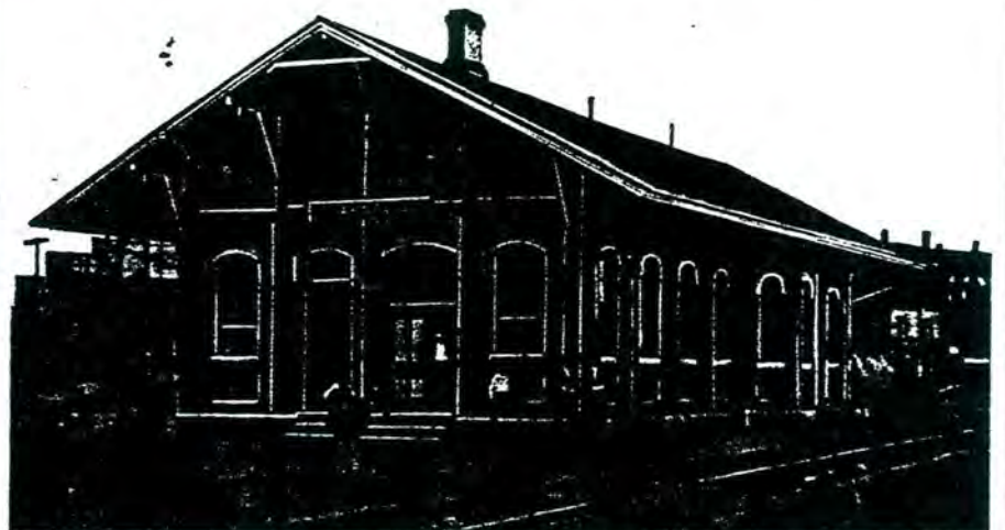
PRR passenger station in Carnegie, Pa., circa 1910. The Panhandle main line is on the left. The Chartiers Branch is in the foreground, to the right. (David Damp collection)
