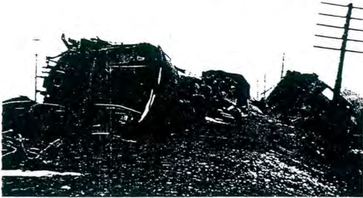
The wreckage of the locomotive and cabin car have been moved off to the north side of the right-of-way.
