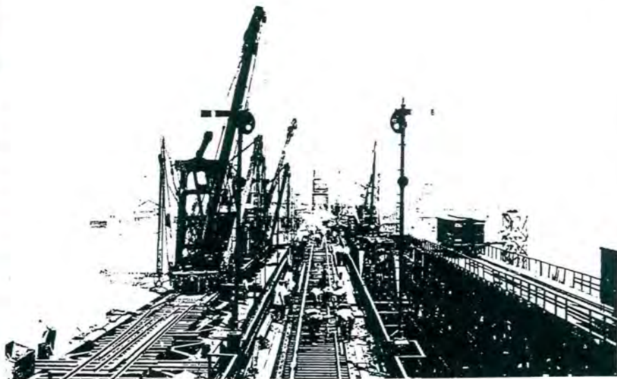
O.C. Bridge construction. Breaking track to move span 10. July 21, 1914.
