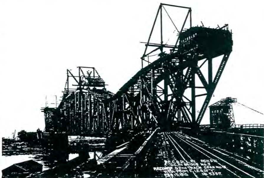
View from the east leg of the "Y", showing construction of the O.C. Bridge, February 15, 1915.
