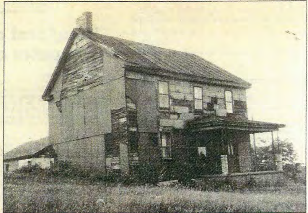
THIS LOG HOUSE stood in Bavington for more than 150 years, until it was removed log by log in 1975.
