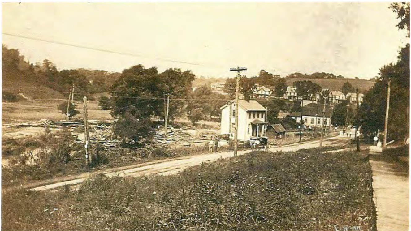
The debris behind the white house is of the Shady Avenue bridge.
