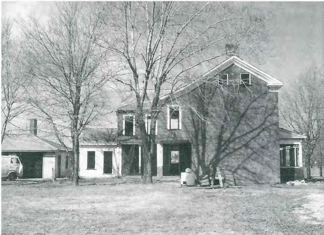
Jesse Ramsey Home Torn down for the Rt. 22 Interchange, Florence
