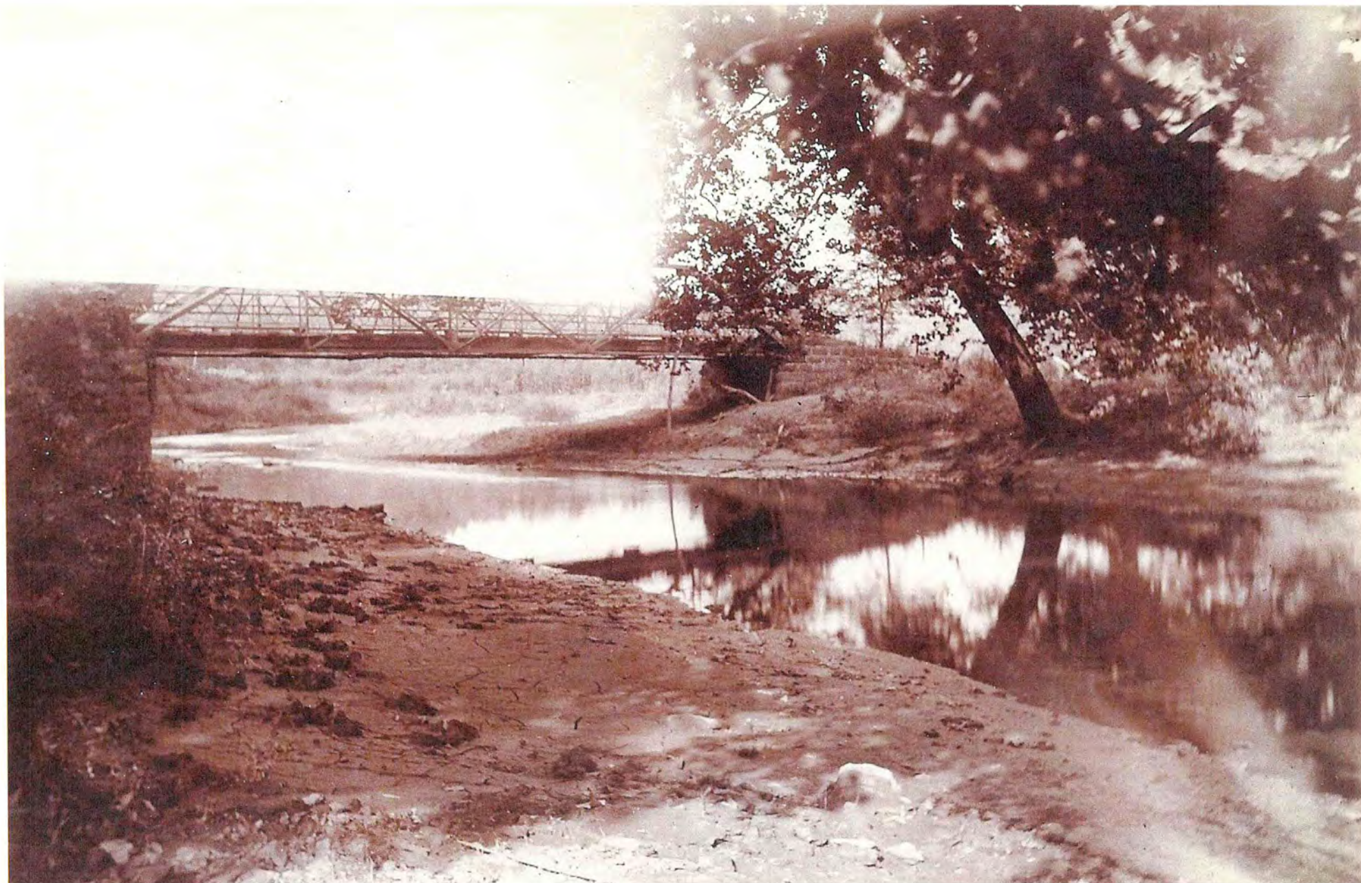
Bridge at Dick Donaldson Farm over Raccoon Creek-Bavington, PA. Photo Courtesy of Roy H. and Olive Scarem
