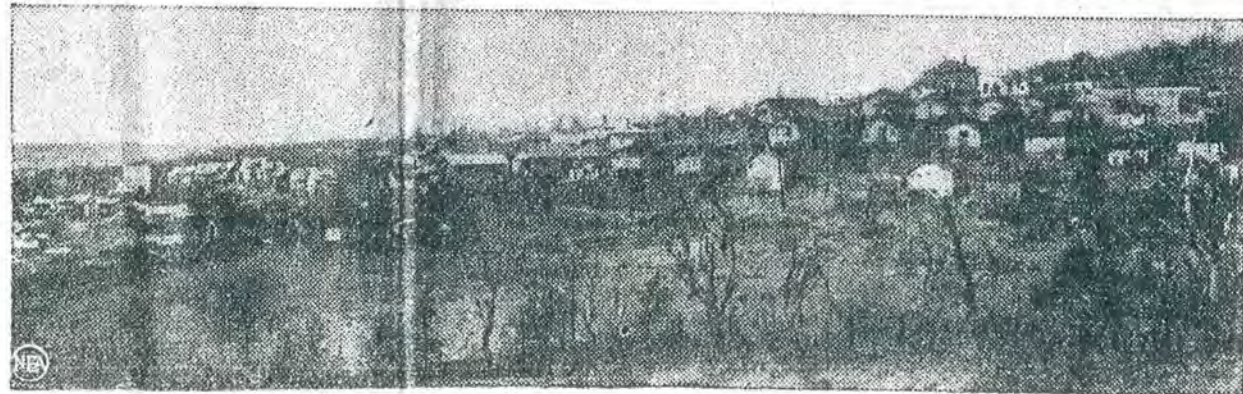
The Town of Langeloth that Gus bought ranges from sagging shanties to a mansion
