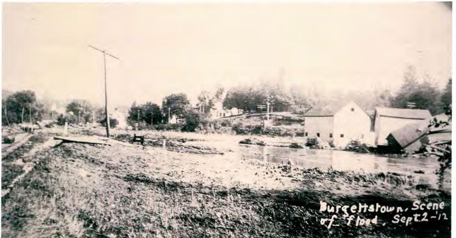
Shady Avenue-Burgettstown, PA Wrecked by September 2, 1912 Flood
