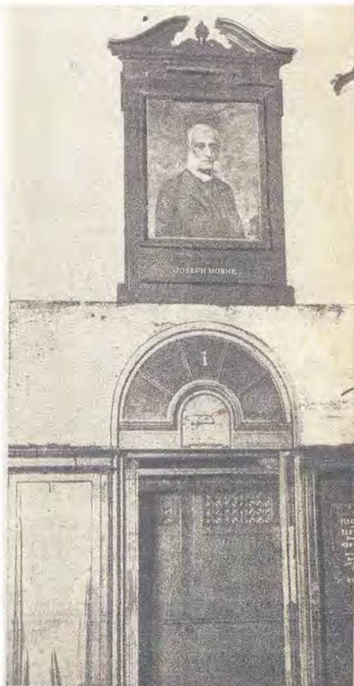
Eighteen inches below the balcony the flood water stopped in the Joseph Horne Company department store, leaving a water mark, on a level with the picture of Joseph Horne, as shown above.
