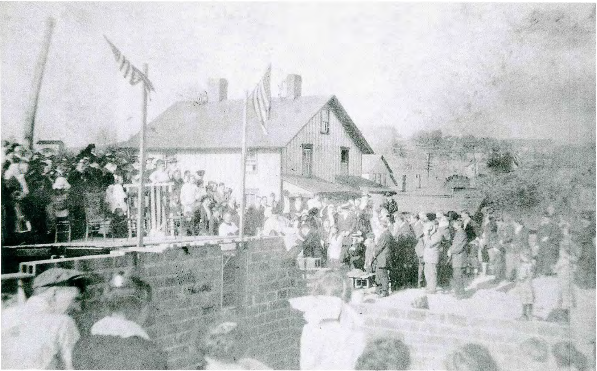
Groundbreaking of St. Ann's Church- Bulger, PA
