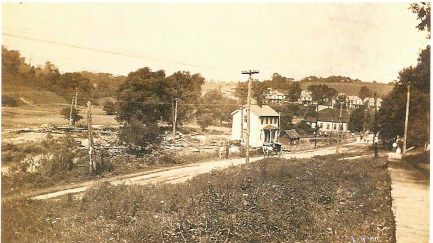
Railroad Tracks Destroyed Near Shady Avenue Bridge Wrecked by September 2, 1912 Flood
