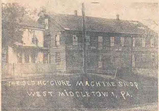
In this building which stood in West Middletown until recent years were manufactured the Ralston horse-powered threshers, widely used in many parts of the country until steam power became general in the later years of the nineteenth century. Robert B.
