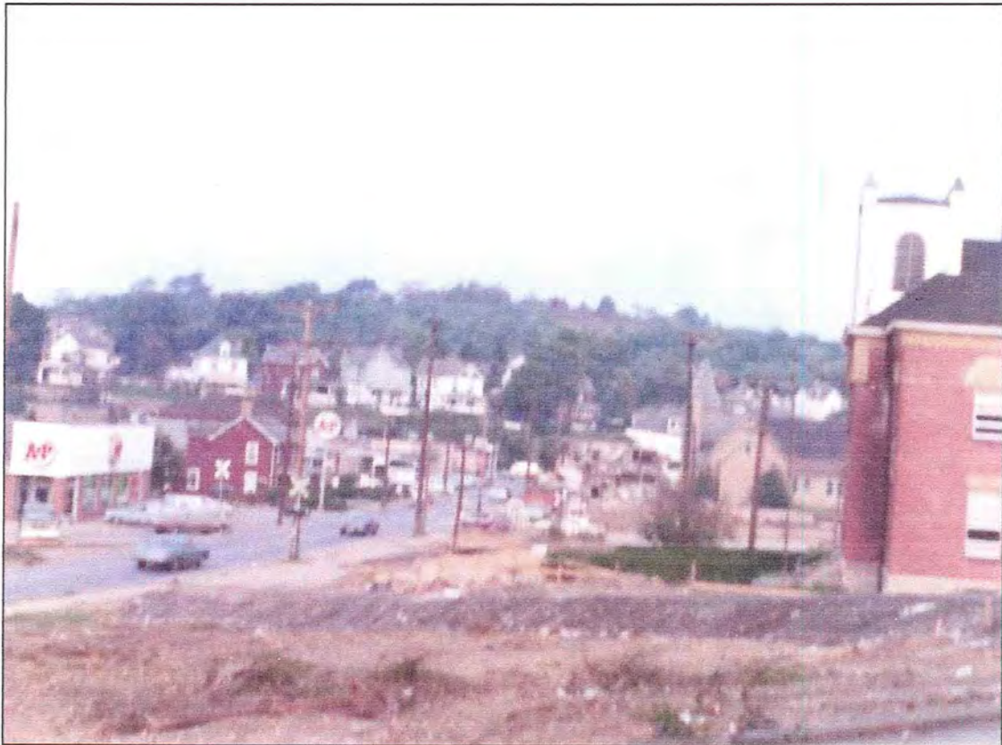
Creating access road in front of Charles Pappas Apartments.
