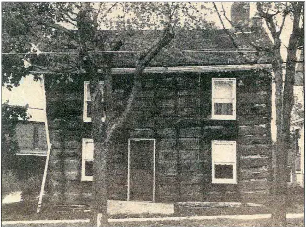
Log House on Market Street, Burgettstown, PA (pg. 4) Restoration 1994
