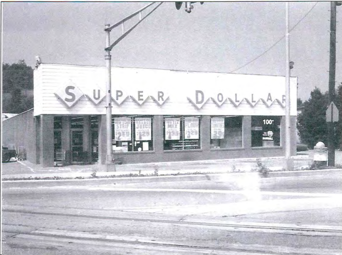
Railroad Crossing in front of Super Dollar, Burgettstown
