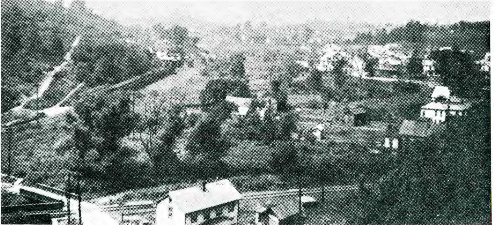
View of Shady Avenue and Dinsmore Avenue, Burgettstown, PA Train tracks to the Patterson Mine Photo taken from Hillcrest Church Tower
