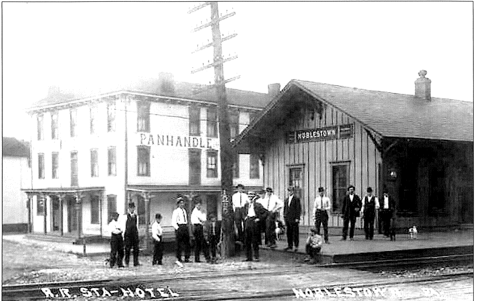
Noblestown Railroad Station and Panhandle Hotel.
