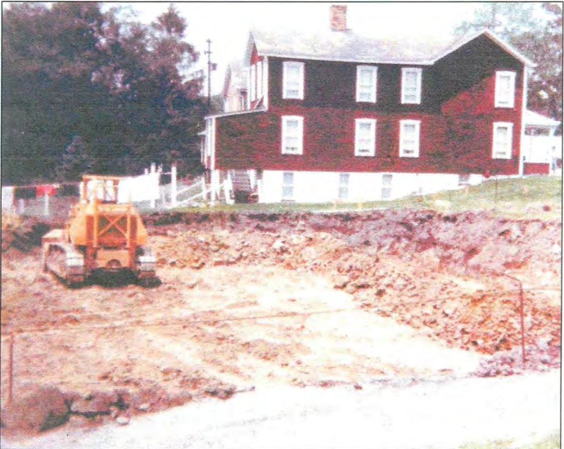
Digging the foundation for Stop & Go-Florence, PA.
