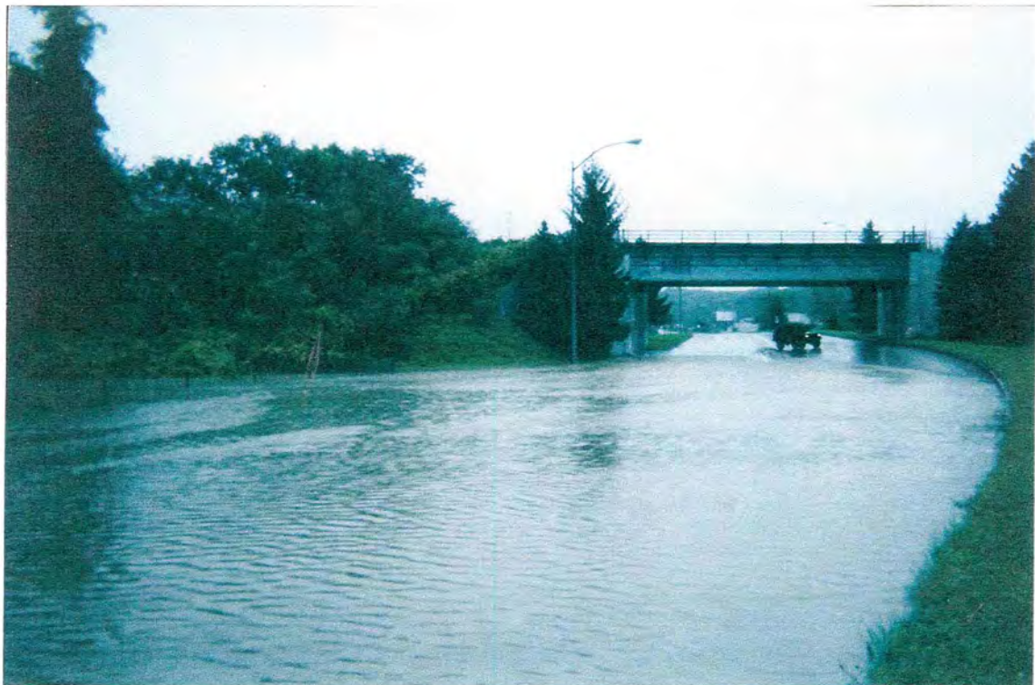
Rt. 18 looking North September 17, 2004 Hurricane Ivan Flood
