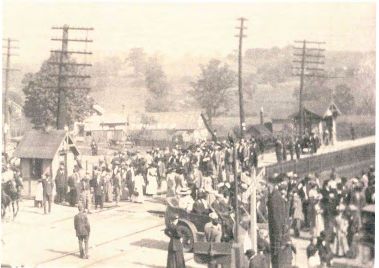
Burgettstown Train Station
