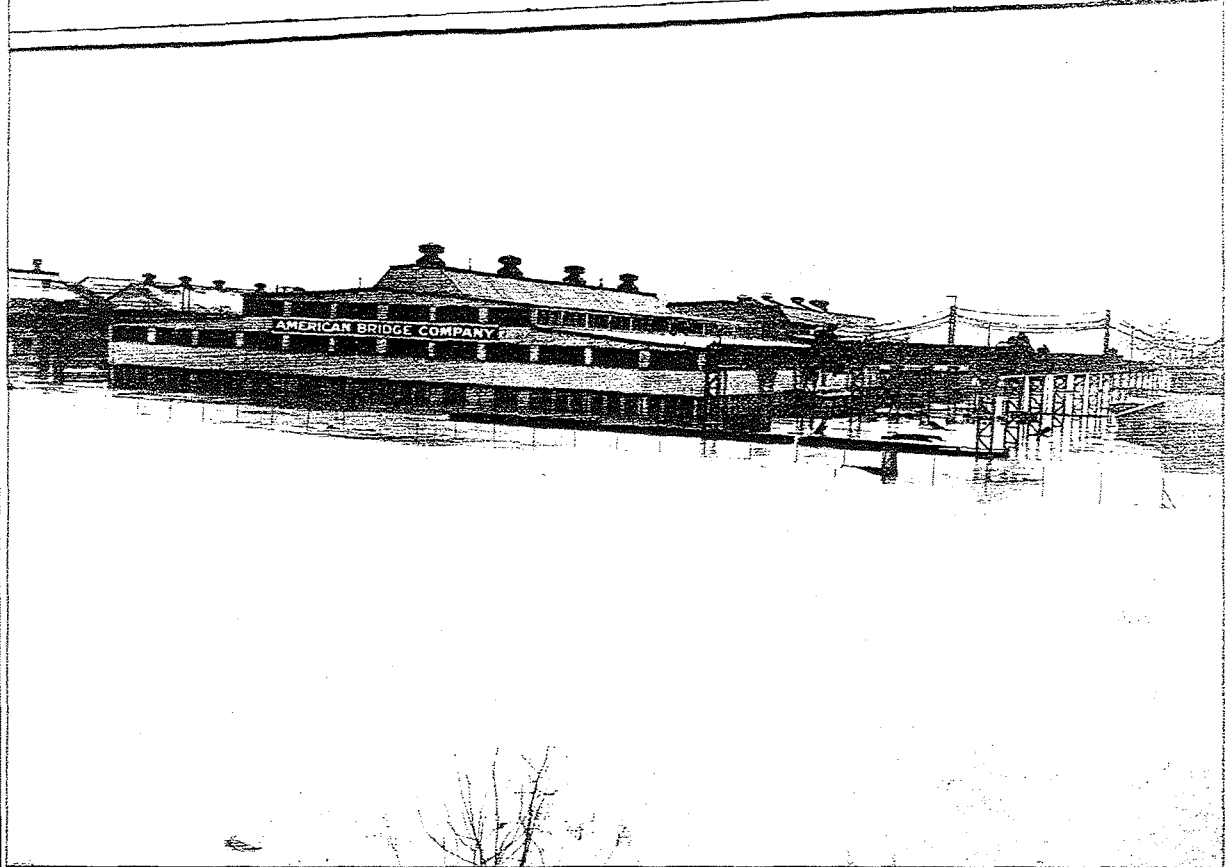
BRIDGE PLANT DELUGED —Swirling flood waters of the Ohio River, racing downward from Pittsburgh, invaded the huge plant of the American Bridge Co. at Ambridge and filled buildings and yards to the top of a fence marking the boundary
