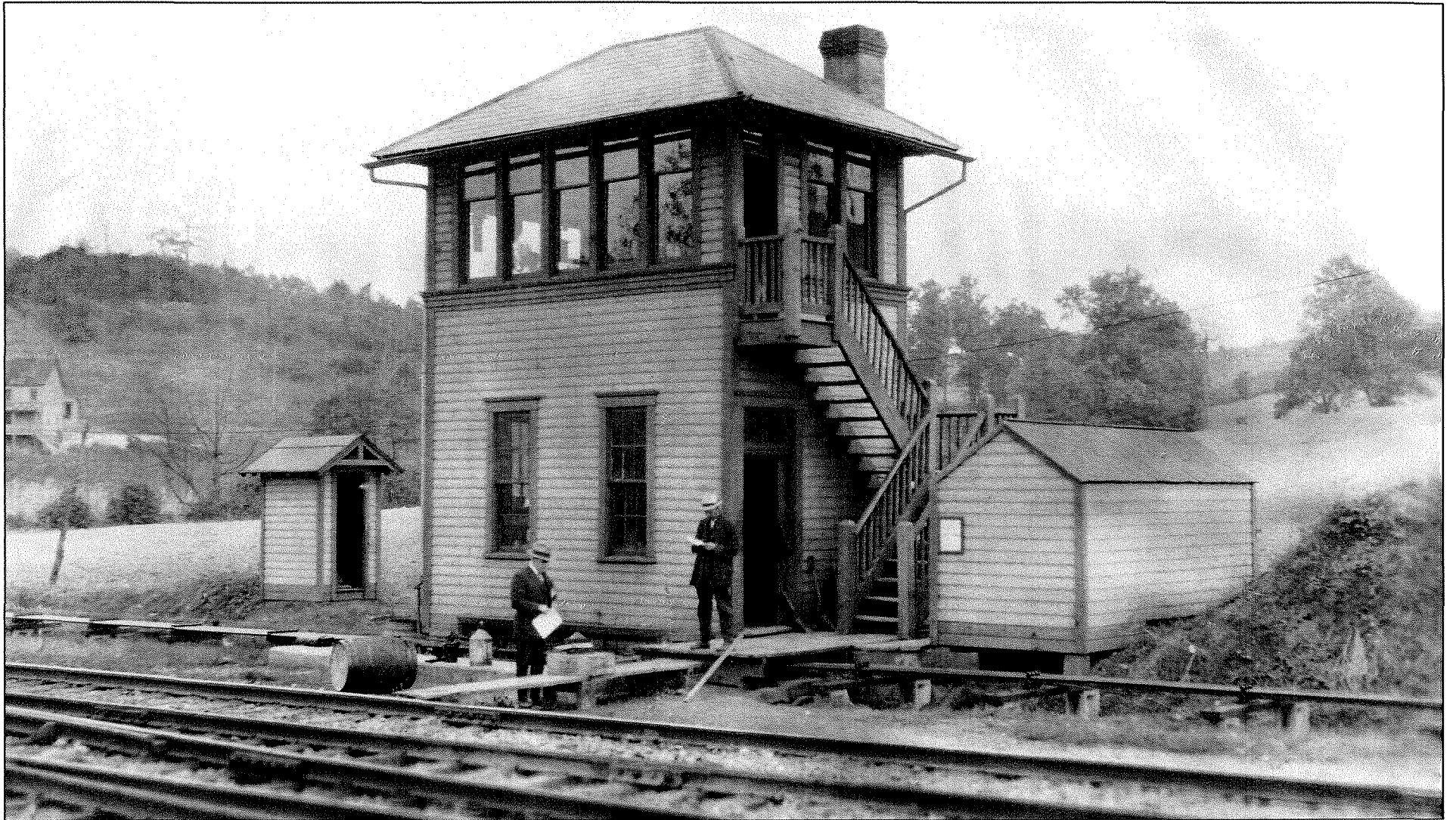
Dinsmore Telegraph Tower-Near Burgettstown, PA
