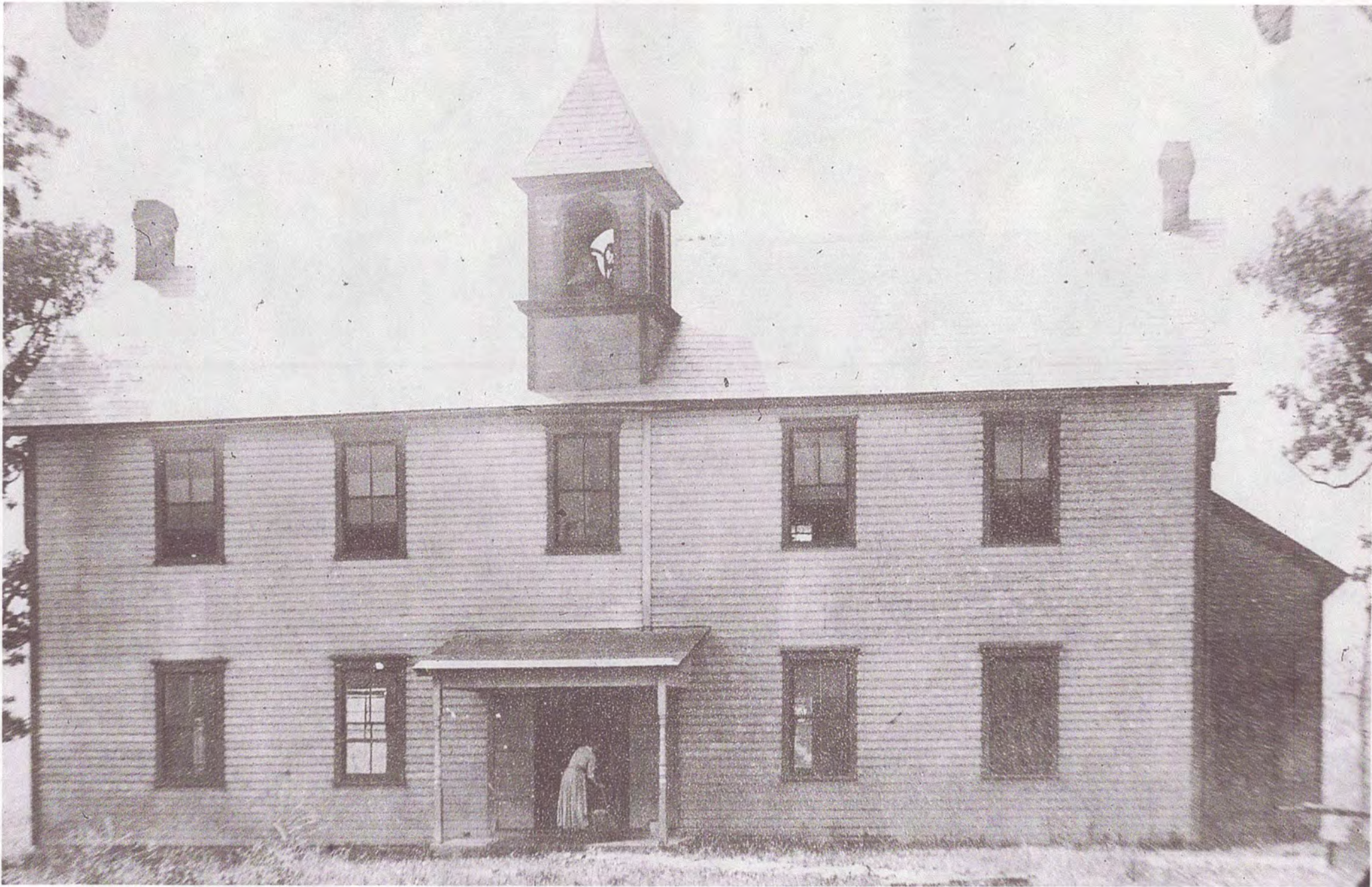
Old Bulger School- Bulger, PA
