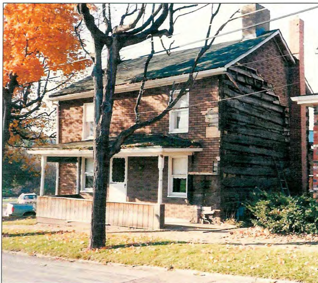
Log House on Market Street, Burgettstown, PA (pg. 1) Restoration 1994
