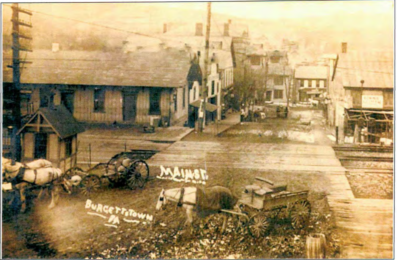
Burgettstown Train Station
