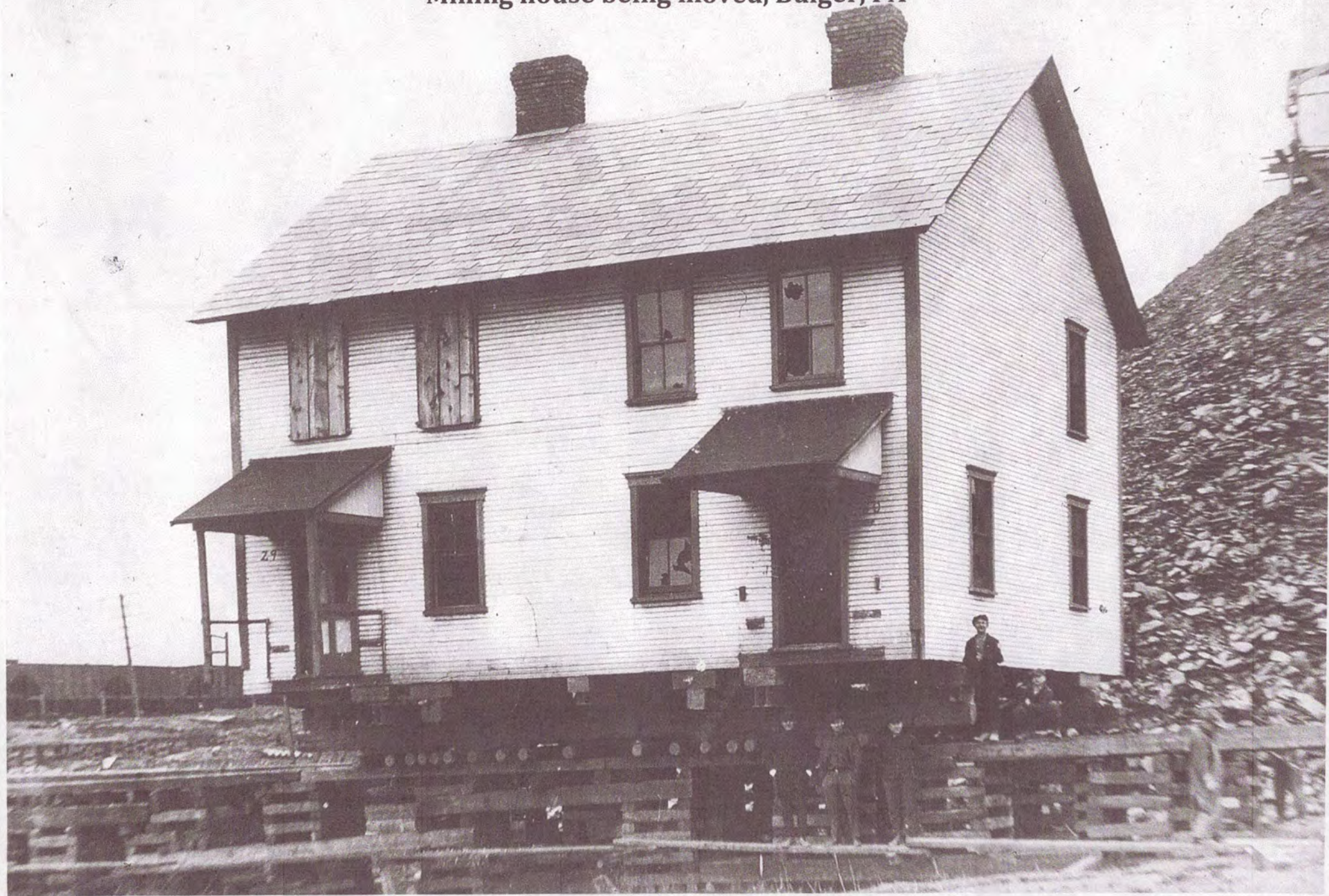
Mining house being moved, Bulger, PA
