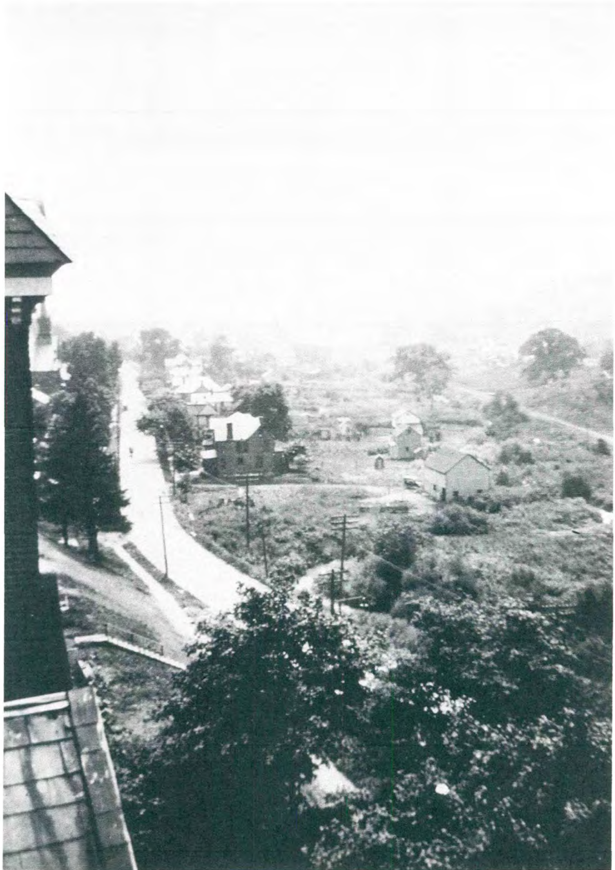
View of South Main Street, Burgettstown, PA Photo taken from Hillcrest Church Tower
