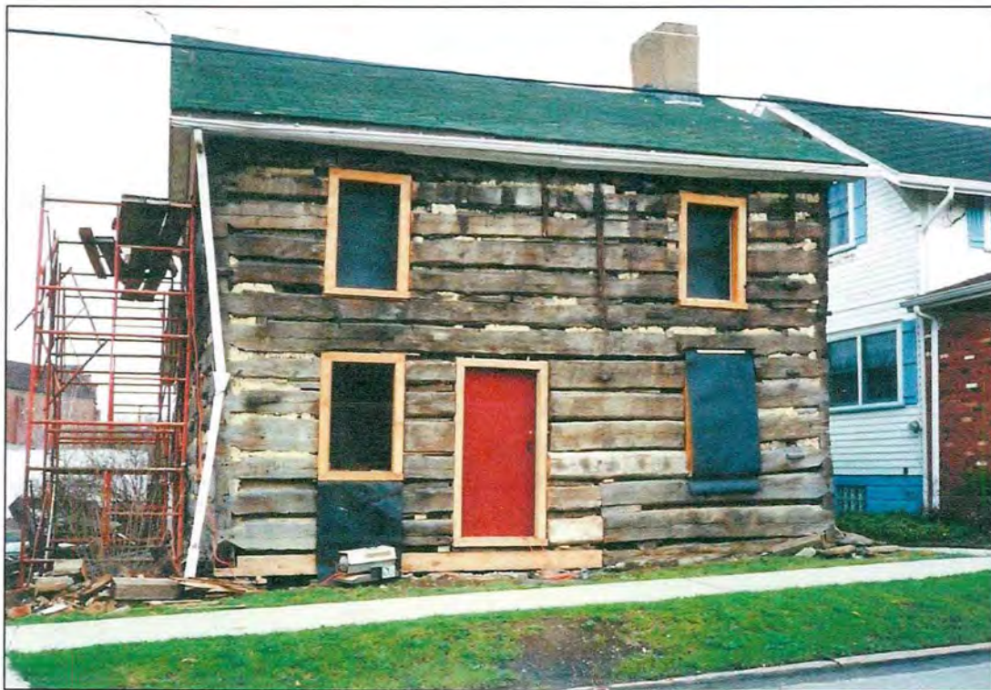
Log House on Market Street, Burgettstown, PA (pg.3) Restoration 1994
