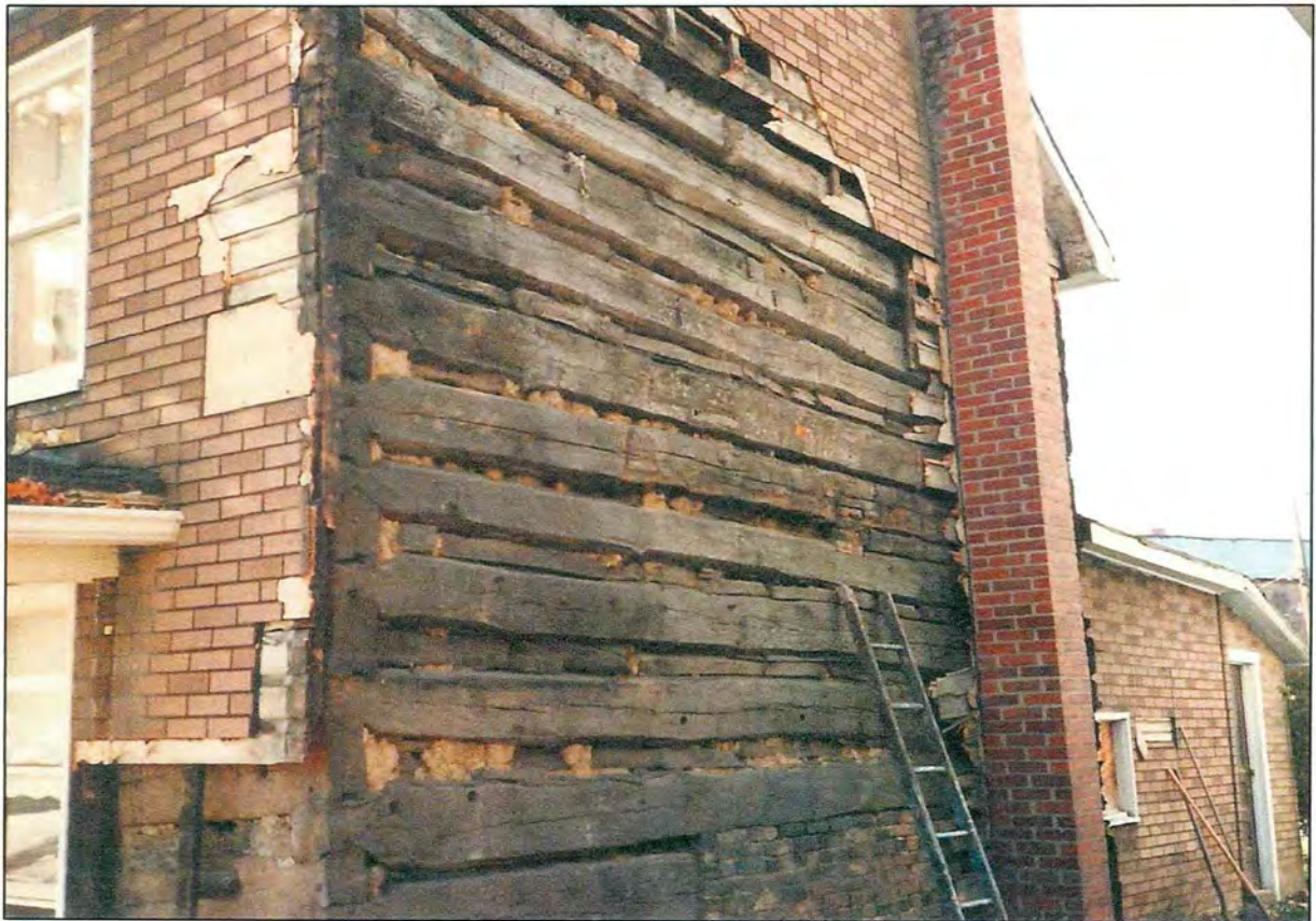
Log House on Market Street, Burgettstown, PA (pg. 2) Restoration 1994
