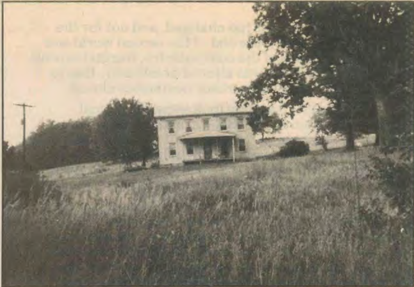
WILLIAM LEE AND his father, Hugh Lee II, built this brick home in 1836. It stands near the foot of the east side of Cross Creek hill, and under the shadow of Quaker Knob, the highest point in the immediate area. This point may be seen to the left of the house. Hugh Lee II died the year after the house was completed. The house is no longer owned by the Lees.
