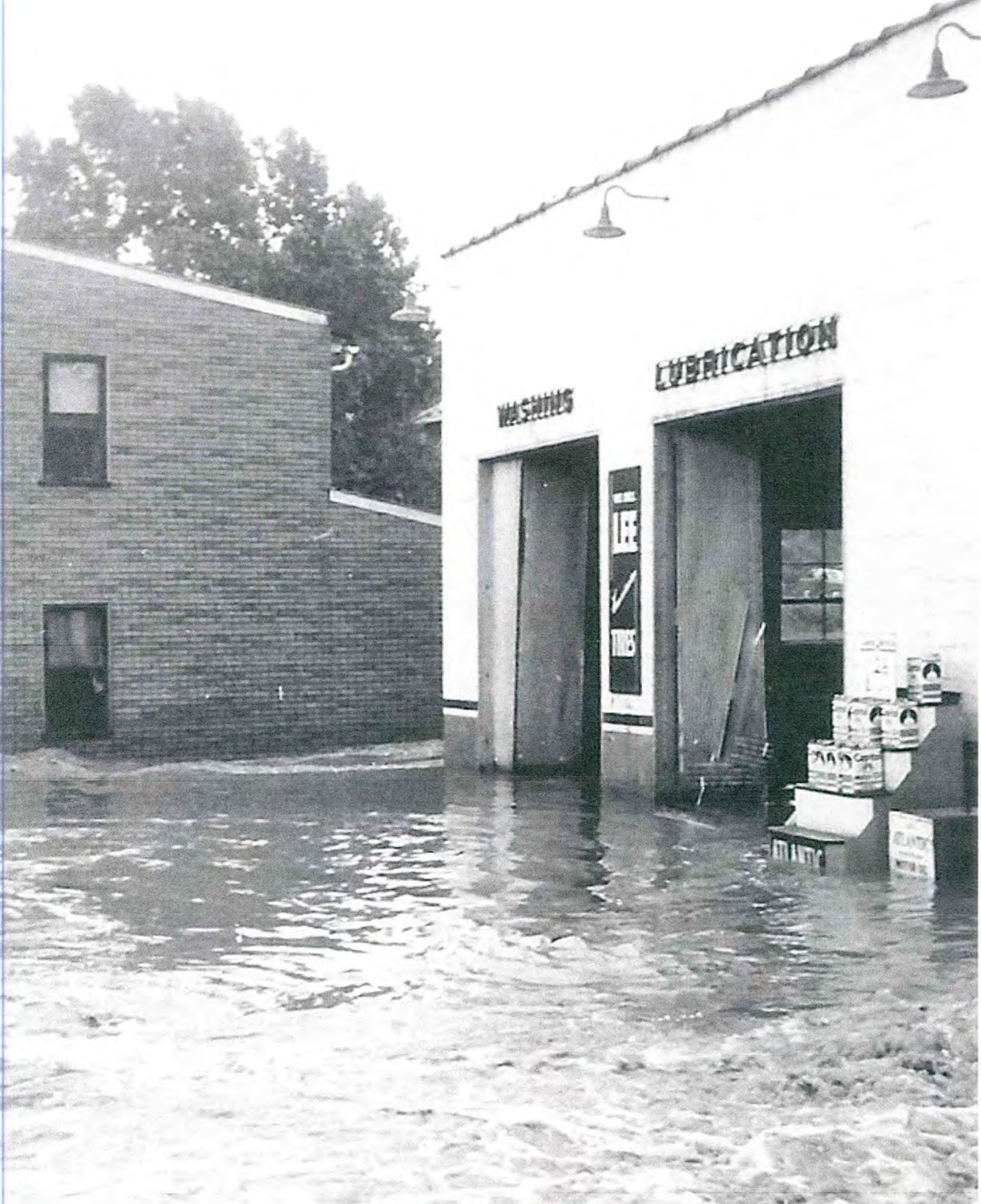
Atlantic Gas Station Bridge Street, Burgettstown, PA
