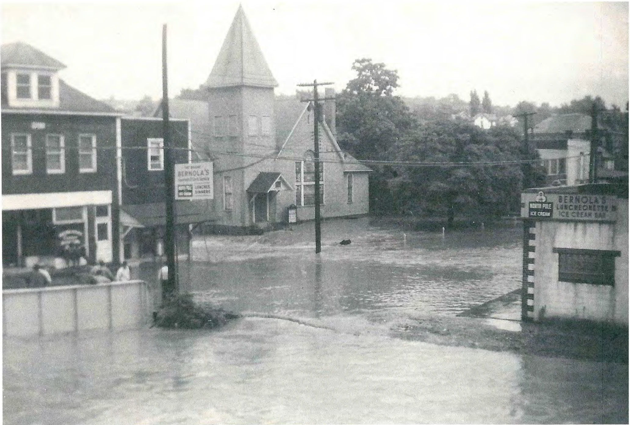
1950 Flood-Main Street, Burgettstown, PA
