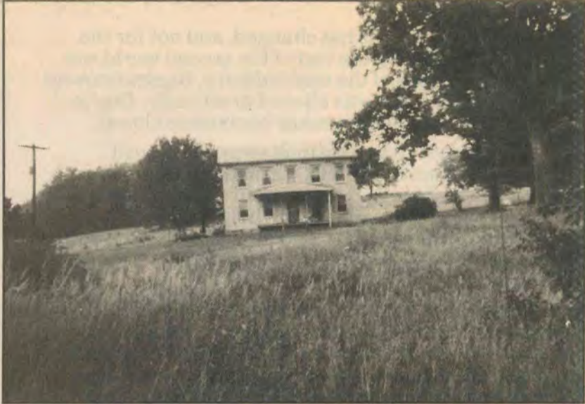
WILLIAM LEE AND his father, Hugh Lee II, built this brick home in 1836. It stands near the foot of the east side of Cross Creek hill, and under the shadow of Quaker Knob, the highest point in the immediate area. This point may be seen to the left of the house. Hugh Lee II died the year after the house was completed. The house is no longer owned by the Lees.
