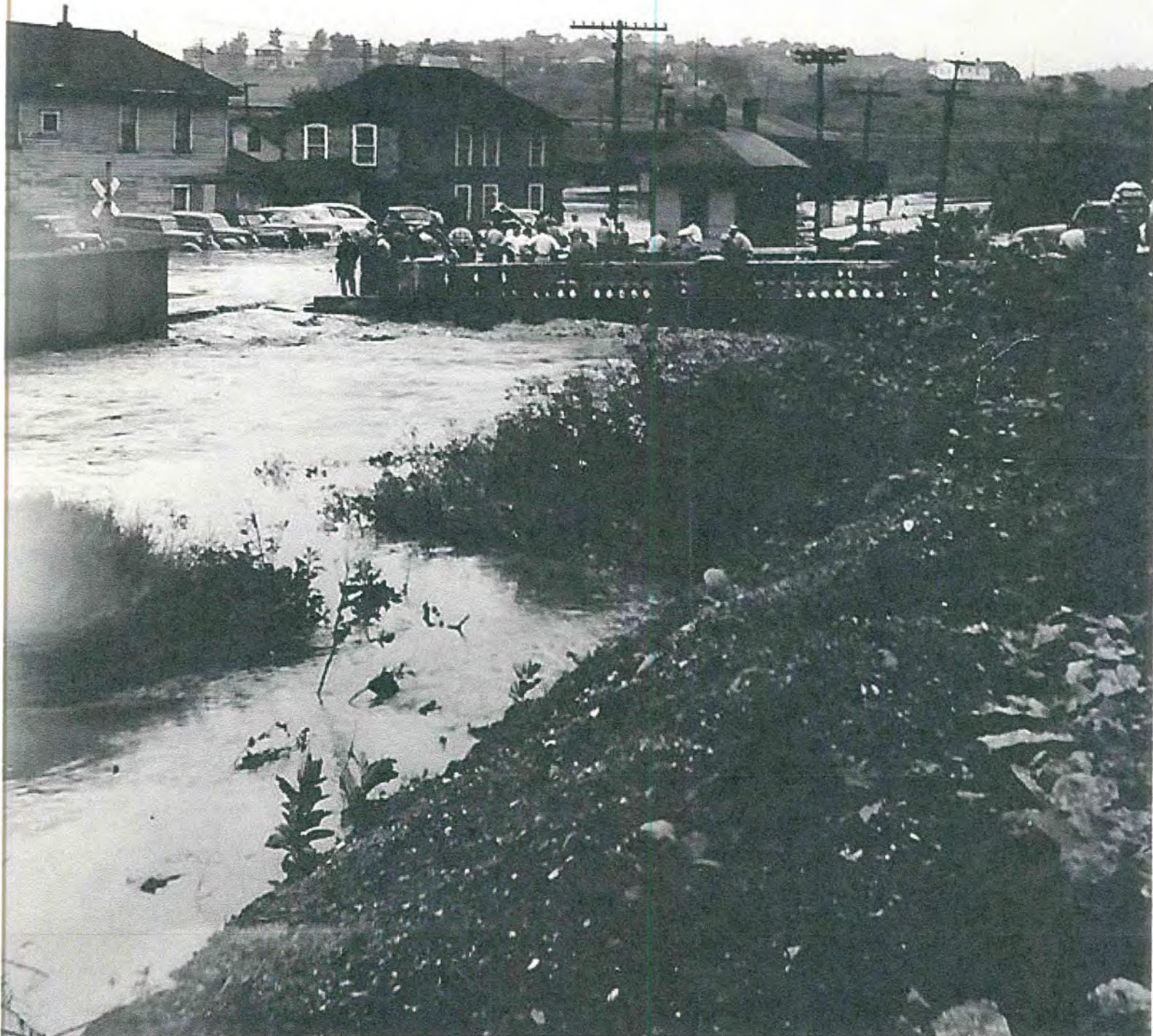
1950 Flood Center Avenue Bridge area-Burgettstown, PA
