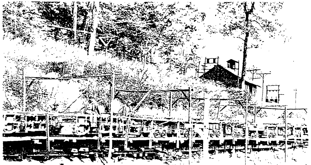
At the Top of the Incline at Louise Mine
