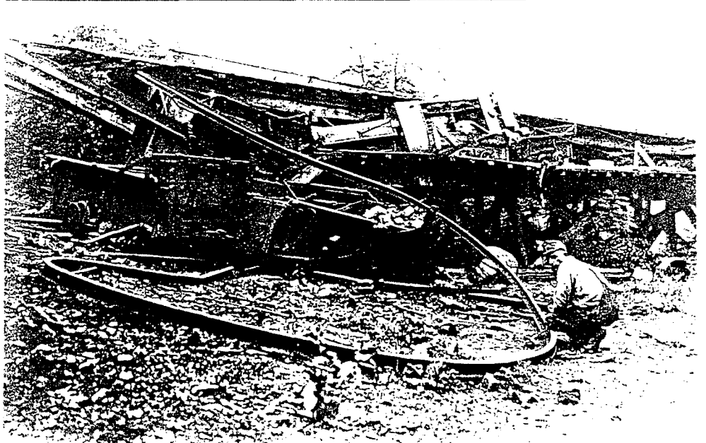
Rails Were Twisted and the Trestle Torn Out
