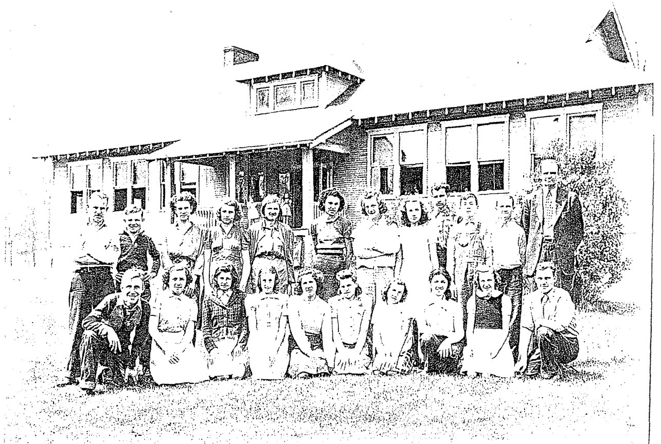
TWO VIEWS OF THE NEW SCHOOL, BUILT IN 1921. SCOTT'S RUN SCHOOL CLOSED IN 1946.
