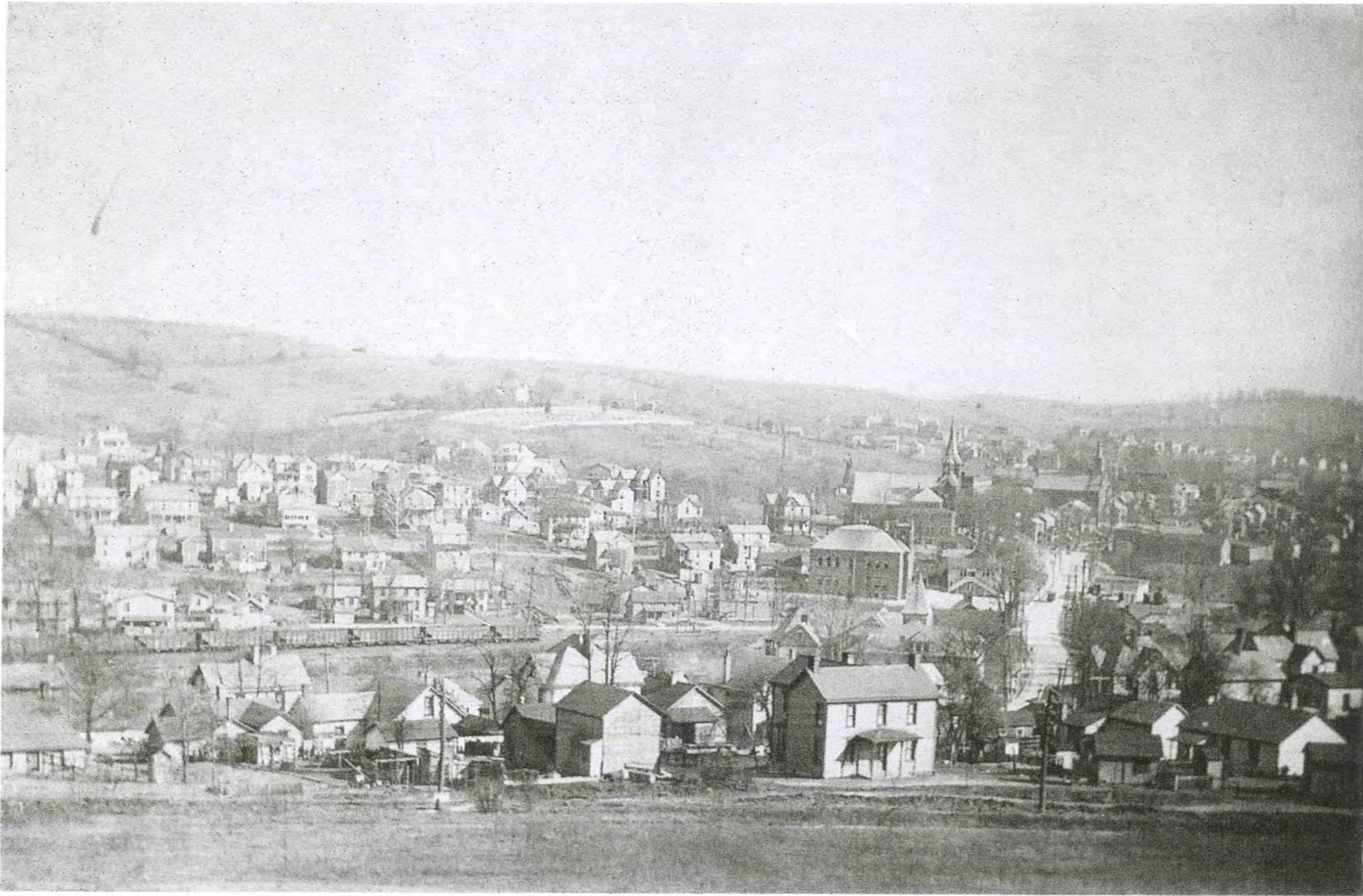
South Main Street Burgettstown, PA
