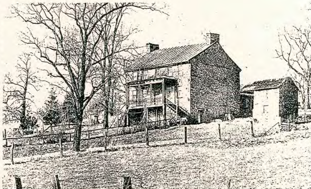
THE PATTERSON STONE house was built in 1794 by William Patterson. This sketch is from Caldwell Atlas, 1876. In 1948, when the house was 154 years old, the end wall crashed to the ground, as was shown in a picture in one of the previous articles.
