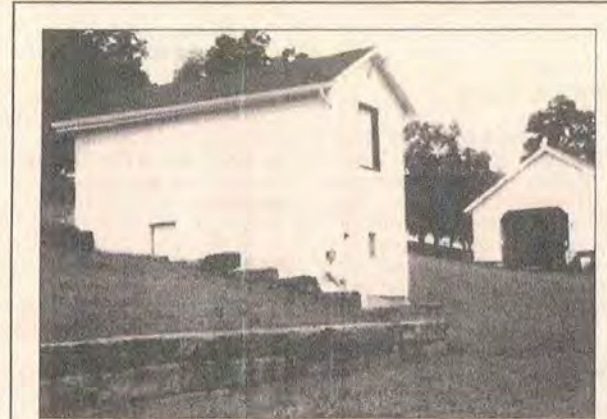
THE SPRINGHOUSE ON the James Patterson farm, owned later by Jacob Mueller and at present by Carrie Paris, is just above the stone wall that extends from the lower side of the house. The wagon shed is in the upper right of the picture. Both were probably built around 1838 when the house was built, and restored in later years. The stone wall is also believed to have been built around the same time.
