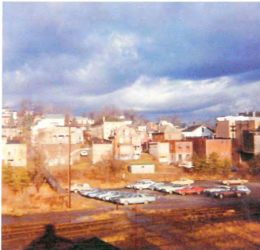
1973-Railroad yard shortly before new by-pass construction
