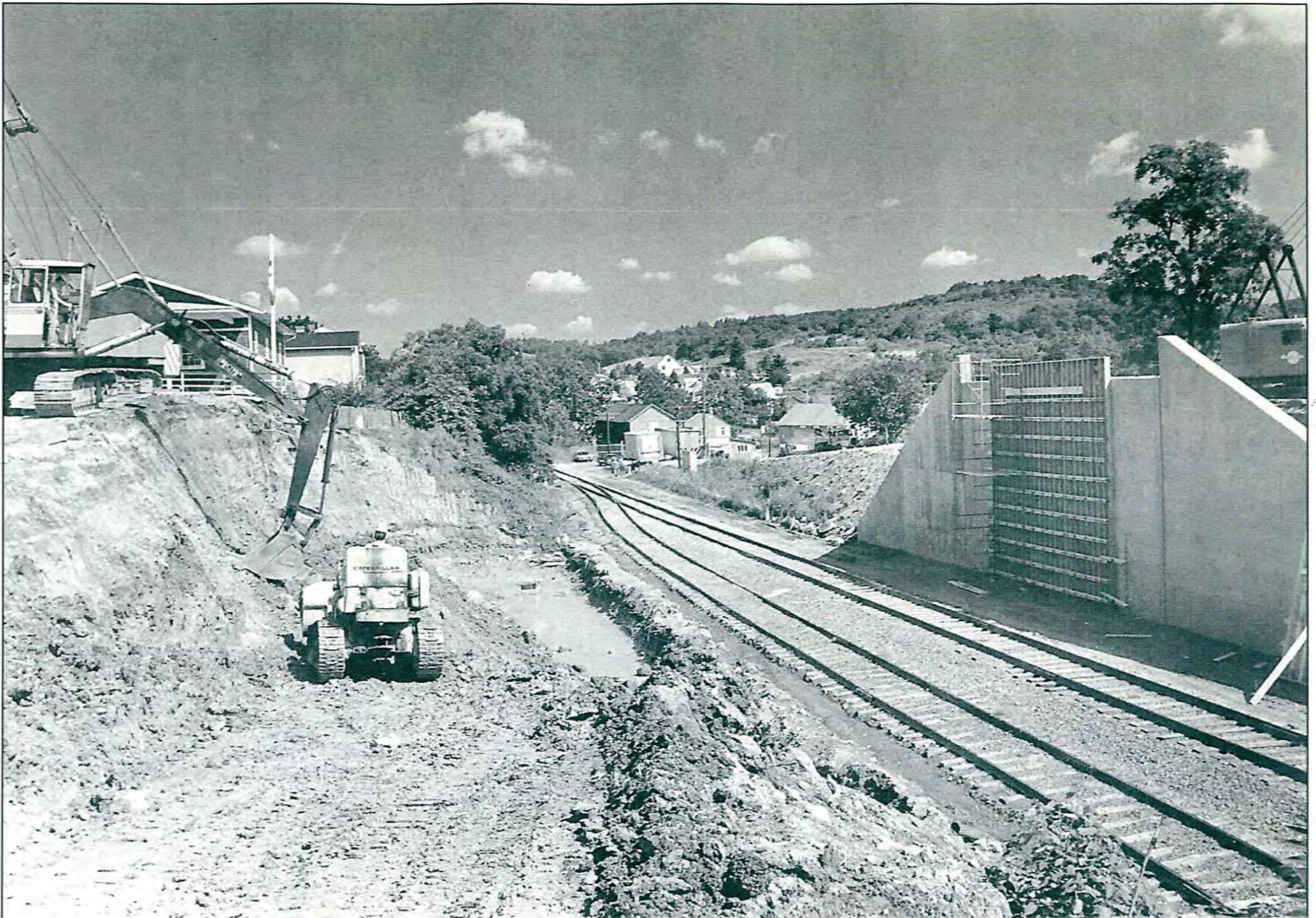
Avella Walbash Bridge Construct-July 1985
