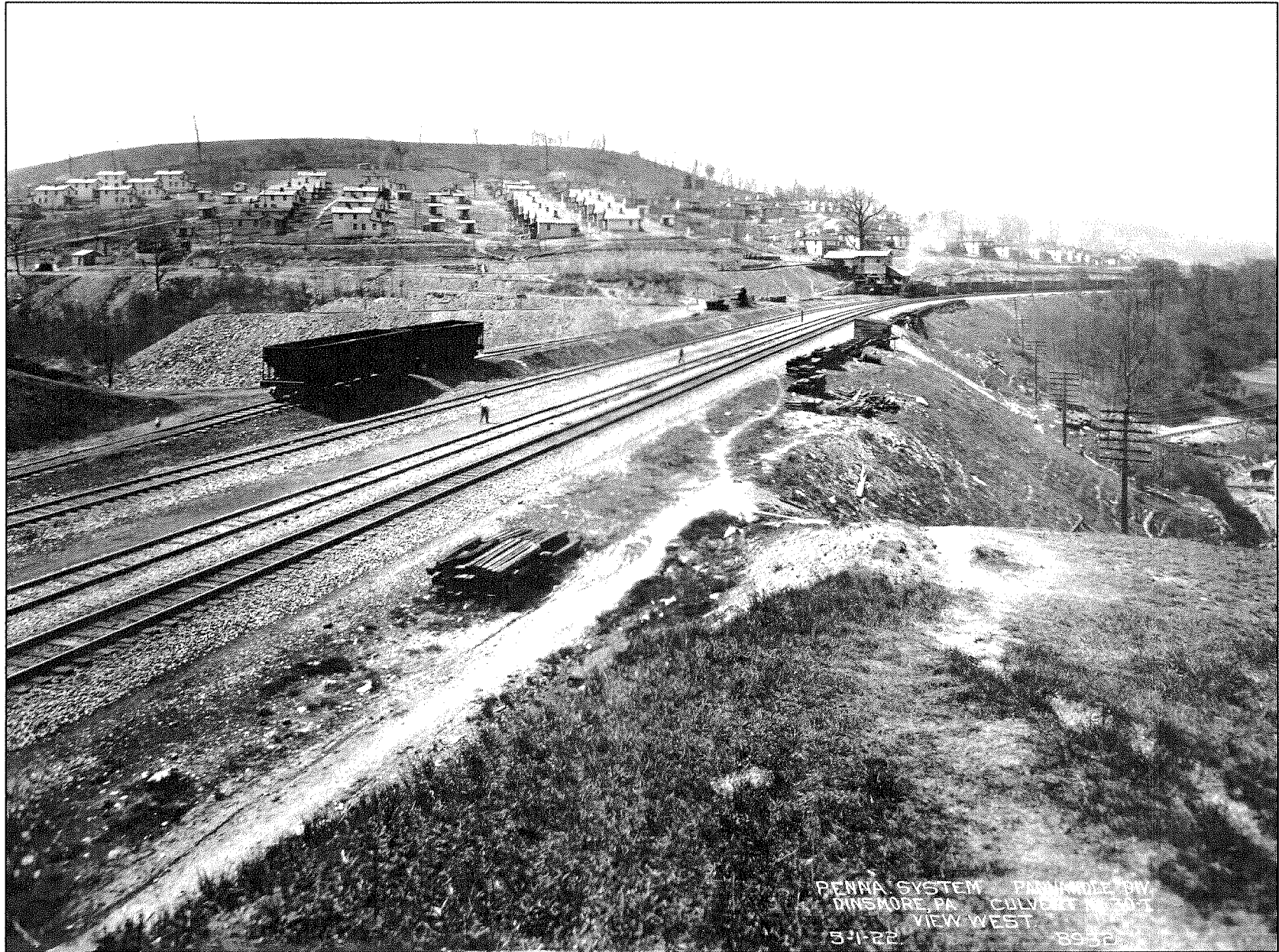
Dinsmore, PA-May 1, 1922 Culvert No. 30-I, View West
