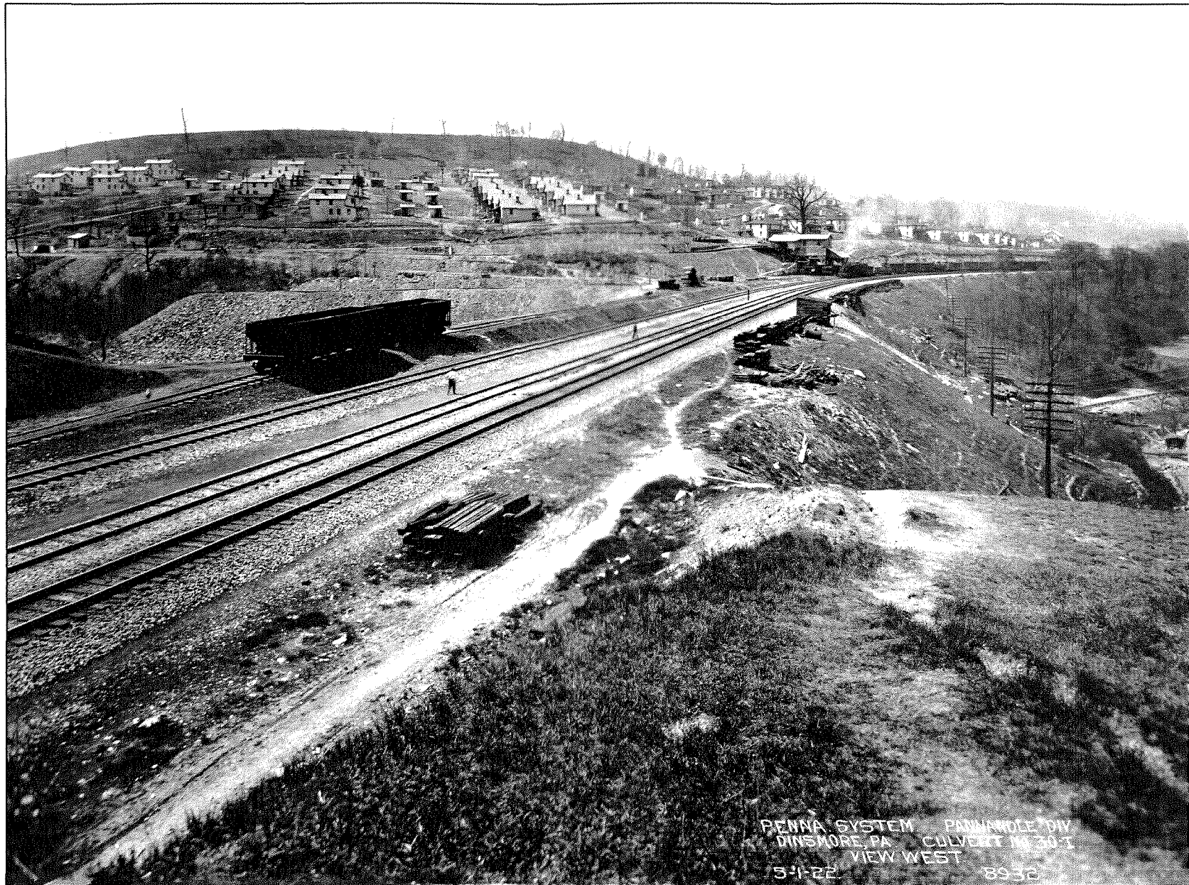
Dinsmore, PA-May 1, 1922 Culvert No. 30-I, View West
