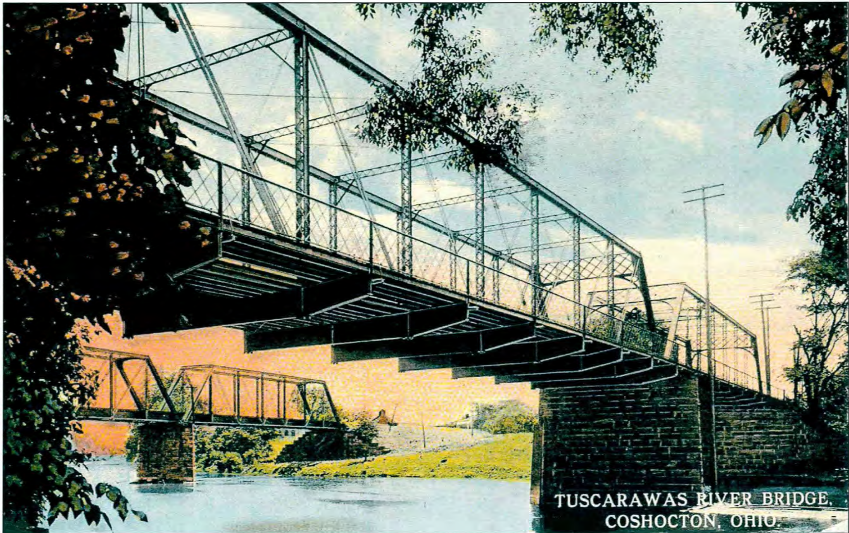
Tuscarawas River Bridge, Coshocton, Ohio-1914
