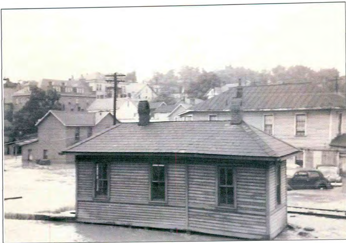
Passenger Station Center Avenue, Burgettstown
