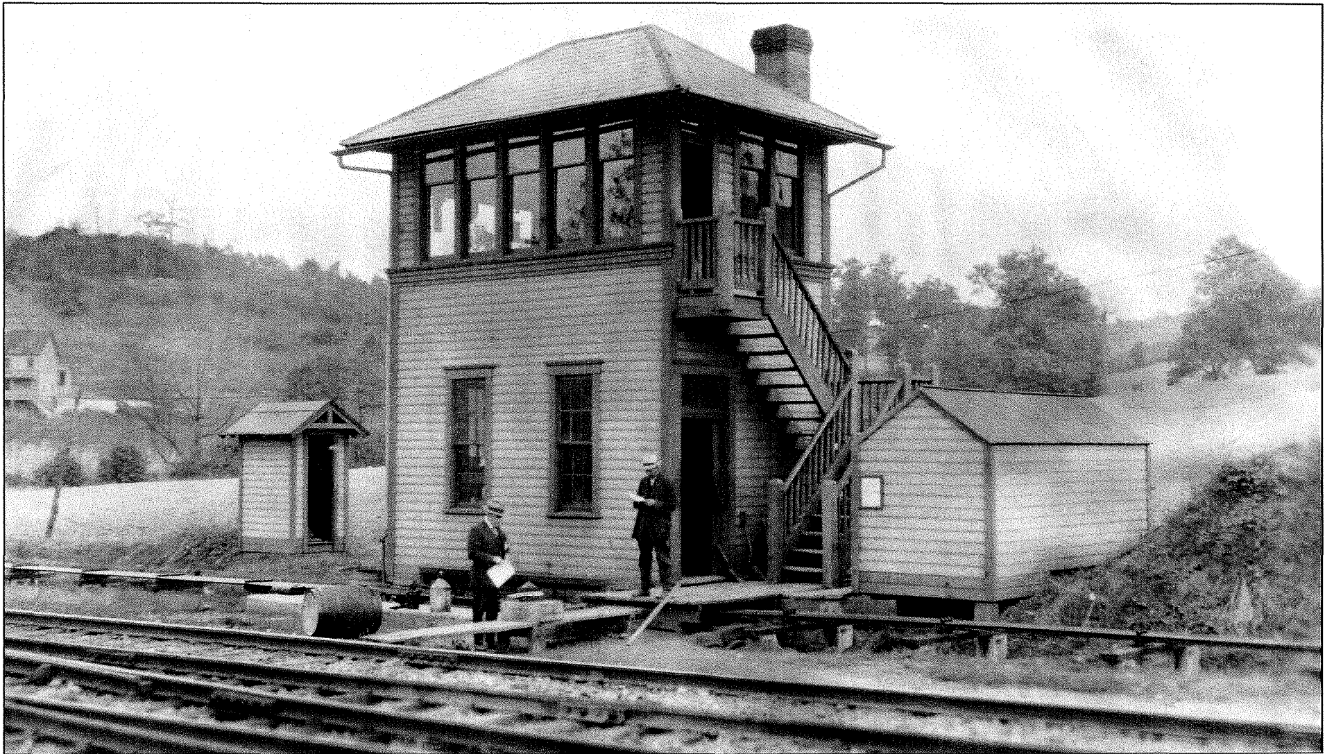
Dinsmore Telegraph Tower-Near Burgettstown, PA
