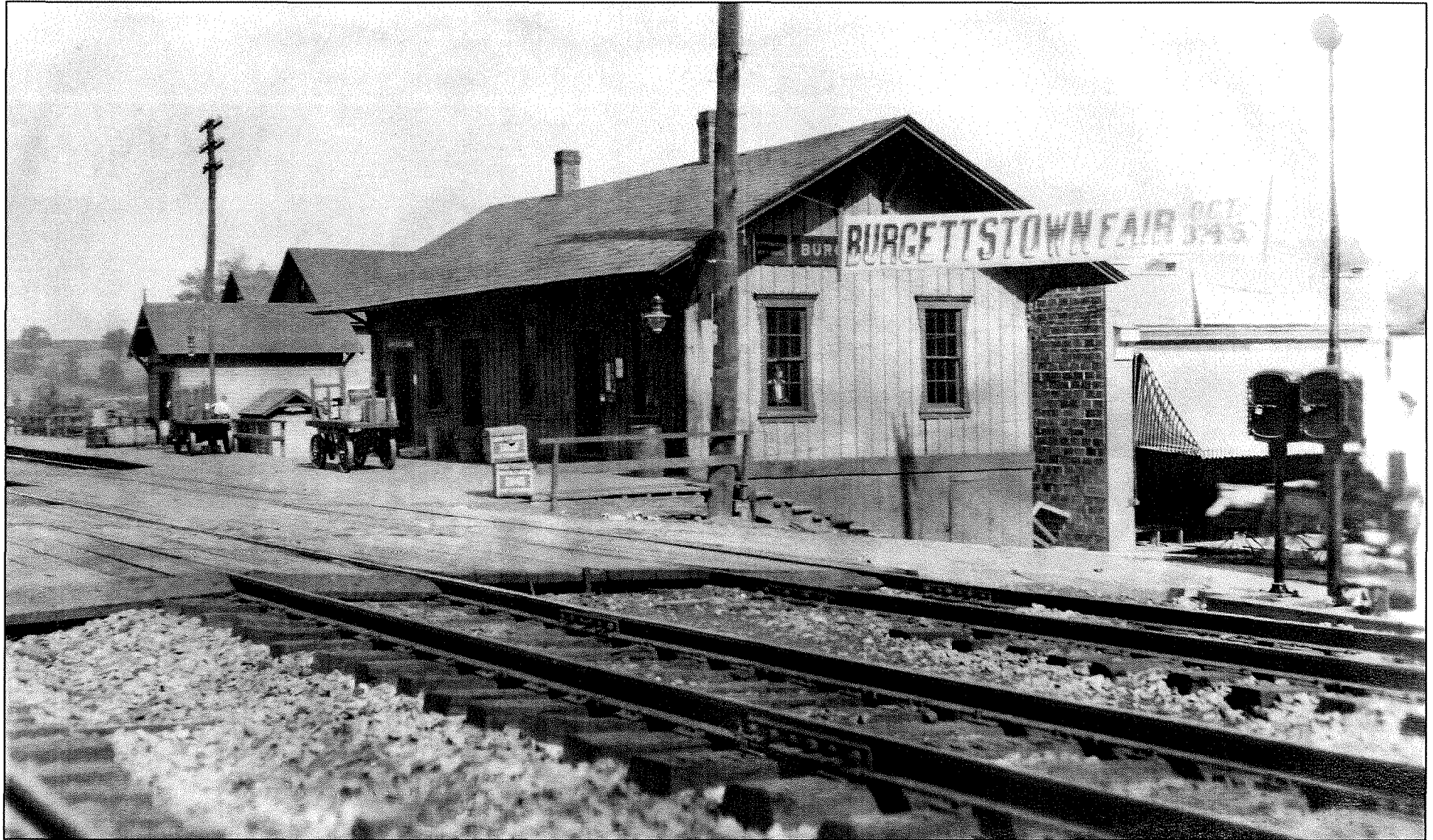
Burgettstown Train Station Welcoming Visitors to Burgettstown Fair
