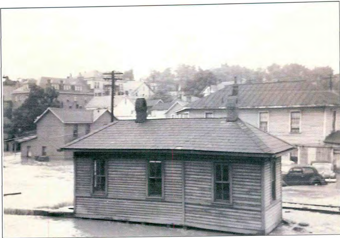
Passenger Station Center Avenue, Burgettstown
