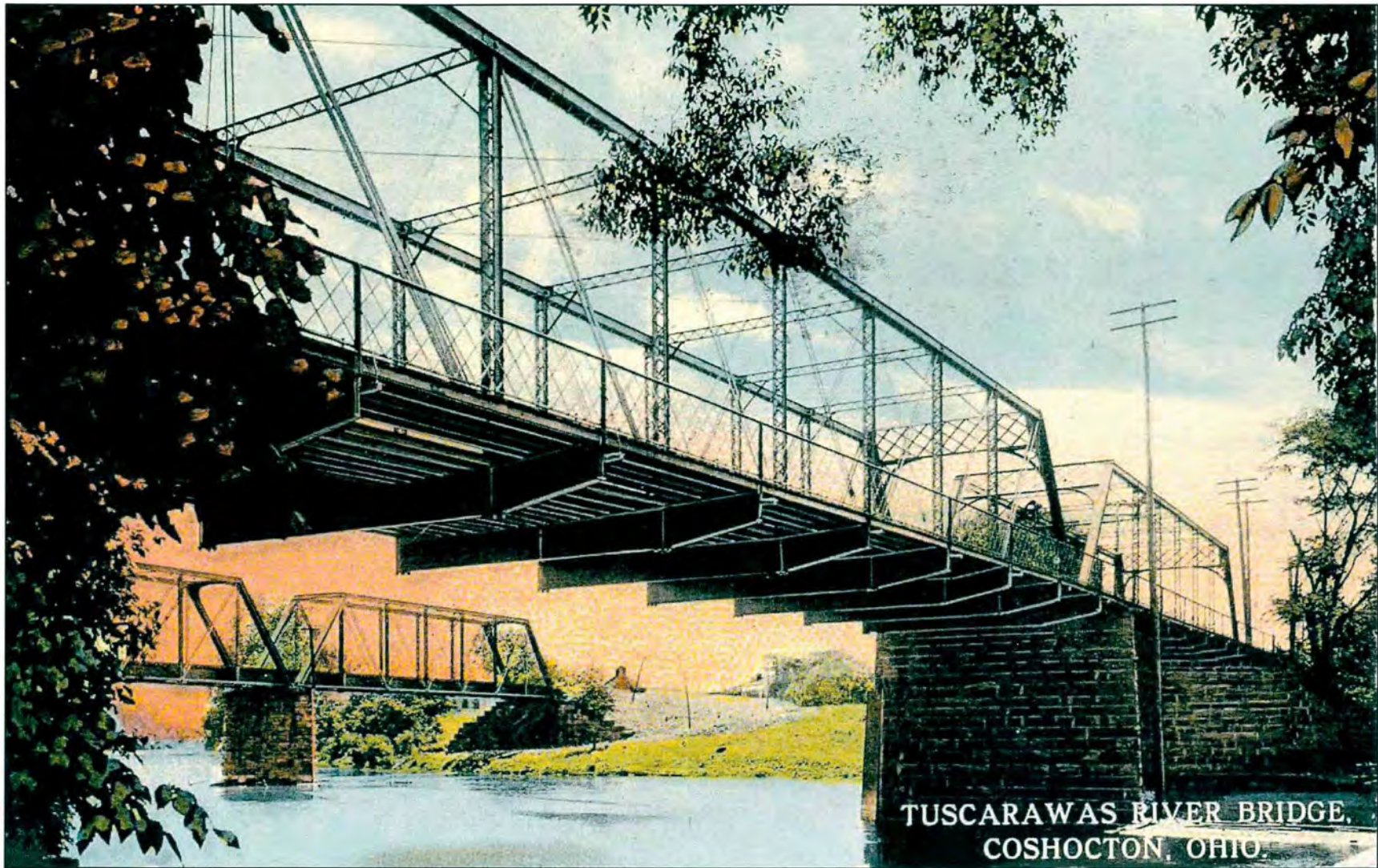
Tuscarawas River Bridge, Coshocton, Ohio-1914
