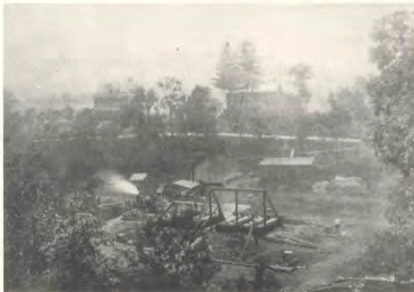
CARNEGIE NATURAL GAS COMPANY - 1915
