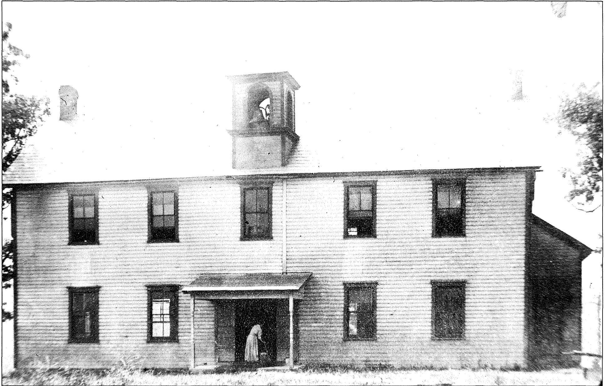
Bulger School-After Remodeling
