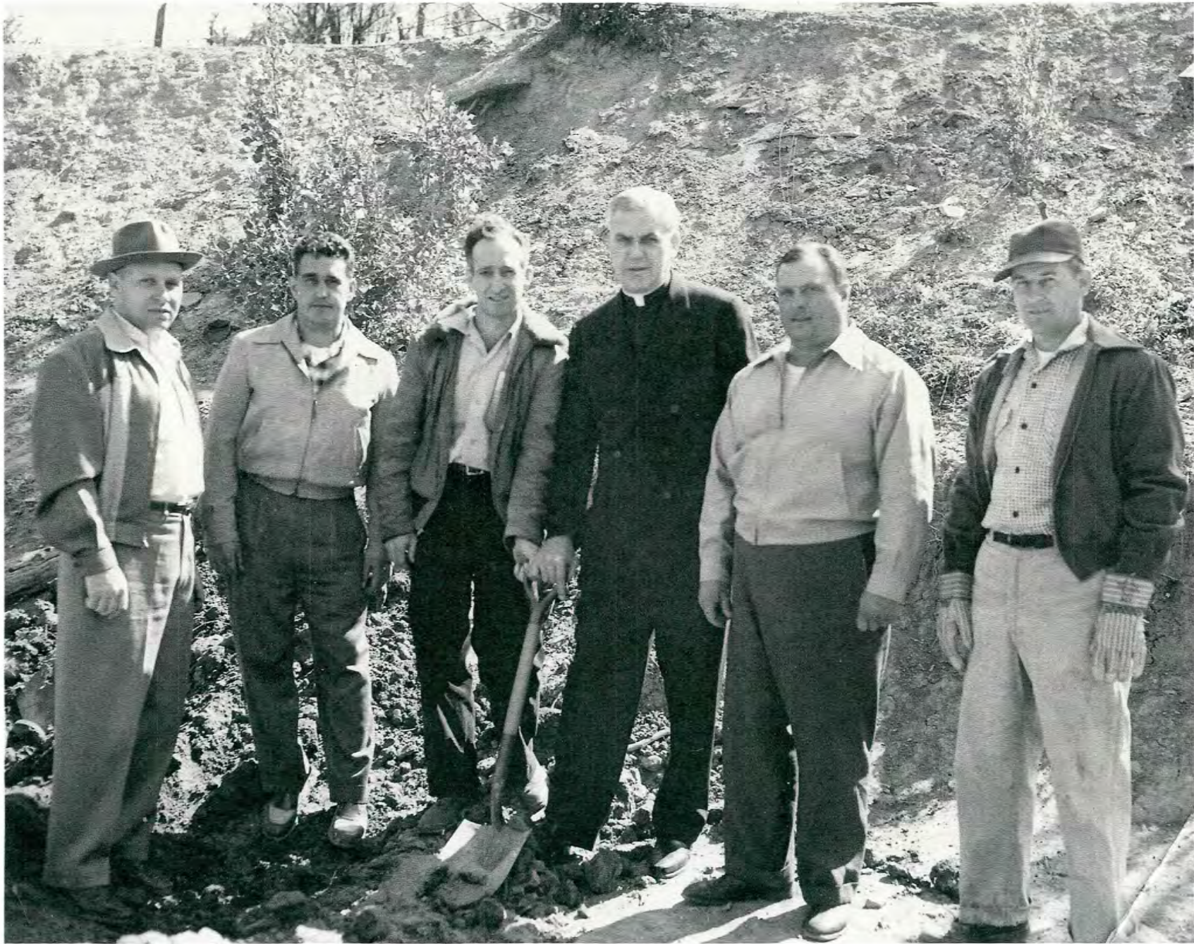
Groundbreaking of Our Lady of Lourdes Playground
