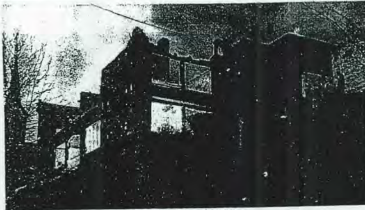
View Of Gutted School Building
