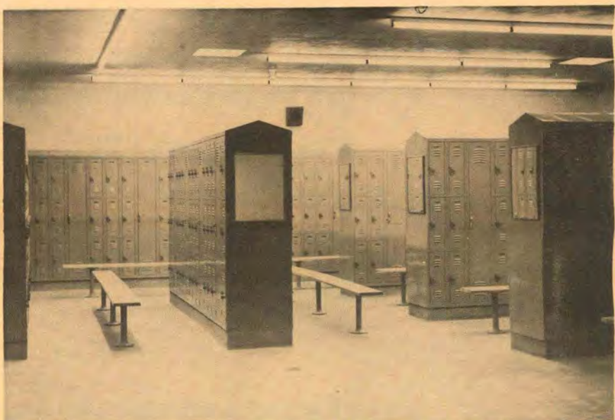
Dressing rooms equipped with individual lockers.
