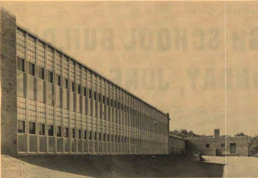
Back view of high school building. Loading docks shown at right.
