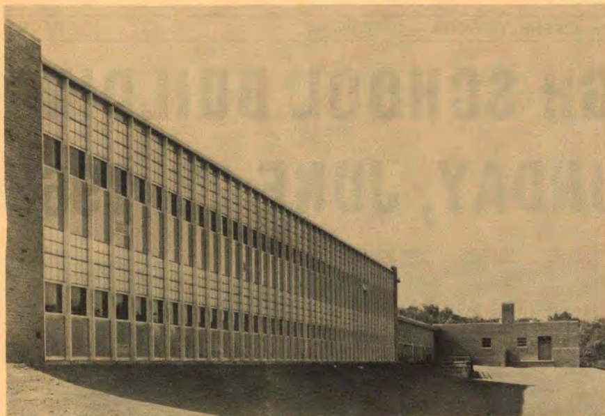
Back view of high school building. Loading docks shown at right.
