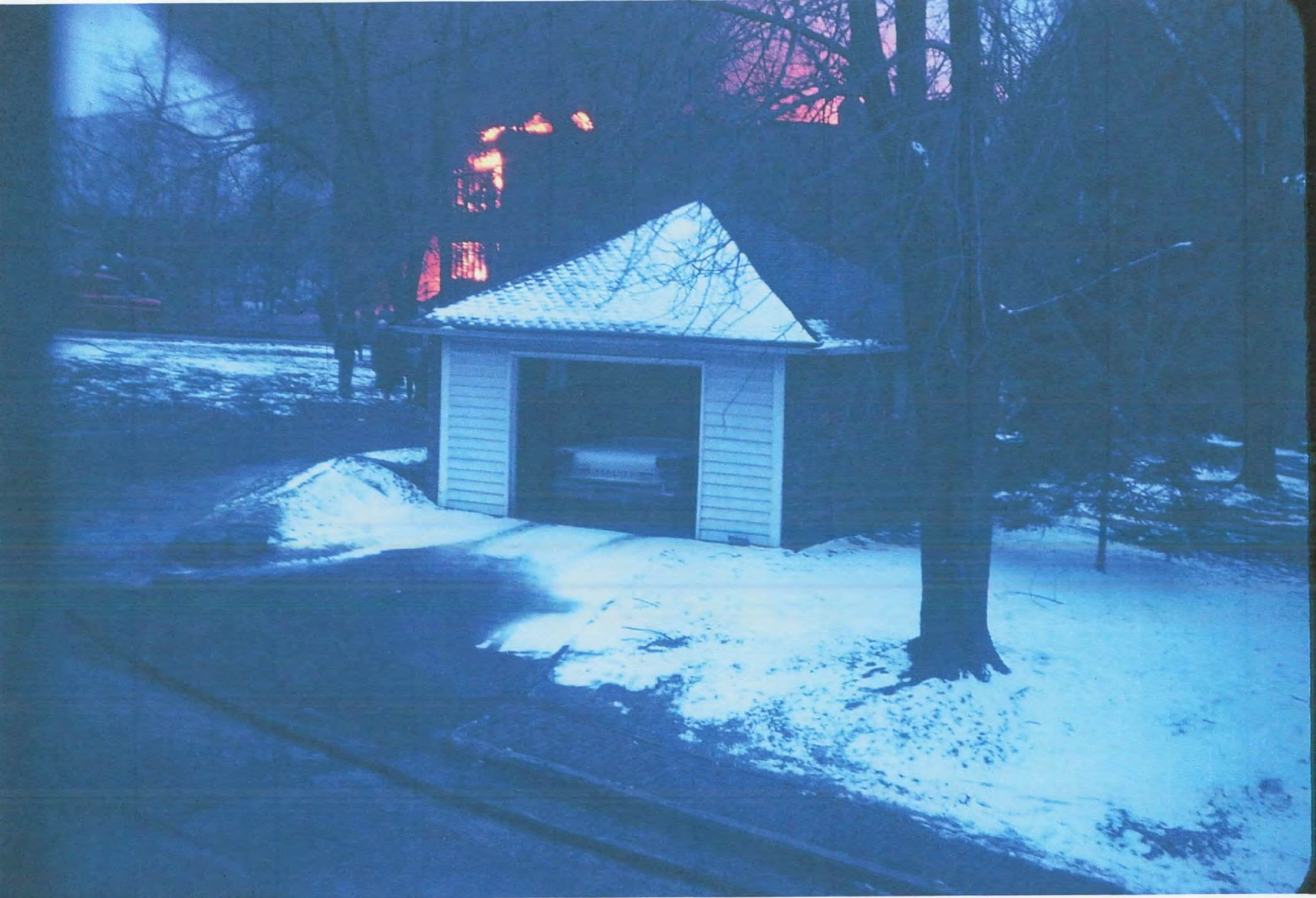
Rear view of Union High School Fire-Burgettstown, PA
