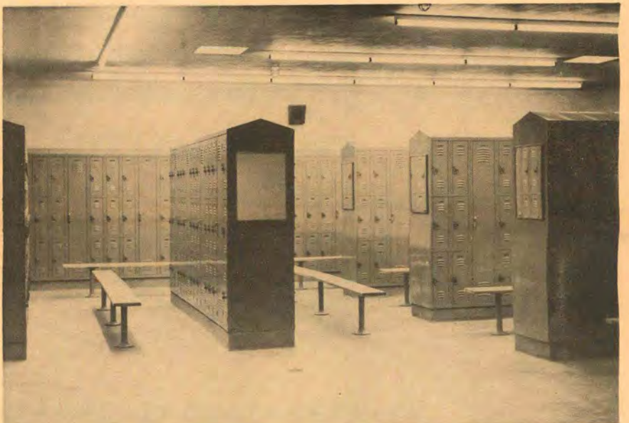
Dressing rooms equipped with individual lockers.
