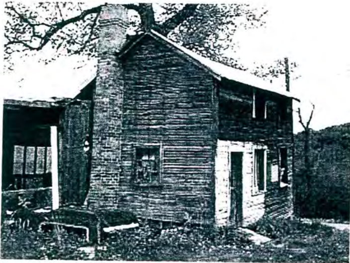
Manchester School in its present location just off Seminary Road near West Middletown. The building has deteriorated into an almost worthless condition.
