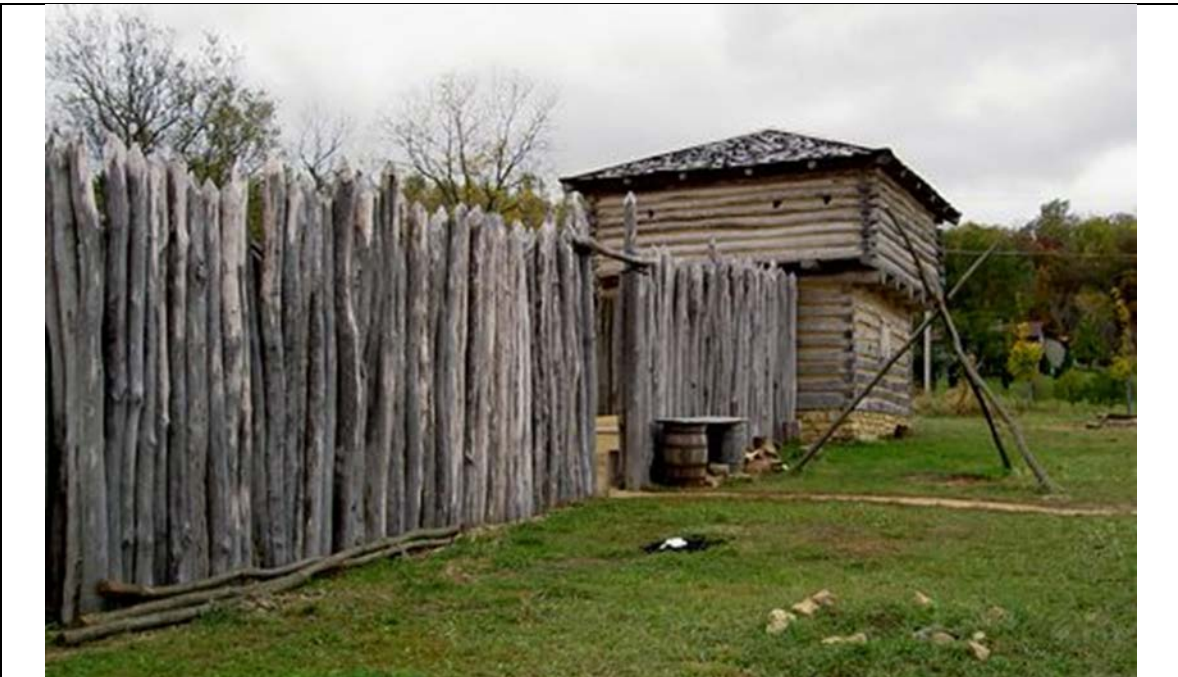
Fig. 3. Reconstruction of Apple River Fort originally built in 1832, now a state historic site located in Elizabeth, IL. Note that the posts appear to be set in the ground and that the second floor of the blockhouse has a clear view of the outer wall of the stockade. The portholes, also called loopholes, were for the flintlock rifles used by the settlers. Photo credit: Wikipedia "Stockade."
