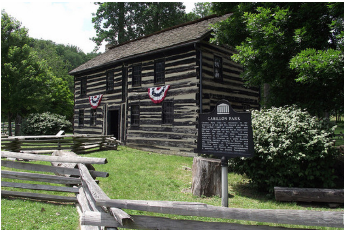
Newcom House was one of the historic buildings in Carillon Park on the 2015 VFA Reunion Tour in Dayton, Ohio
