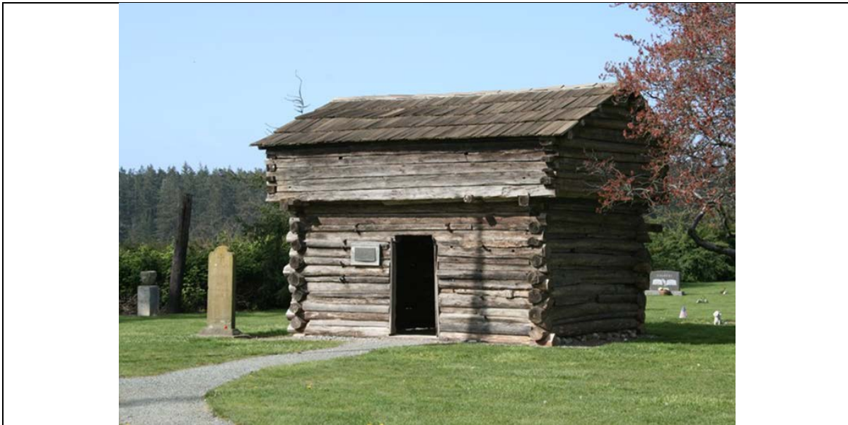
Fig. 5. An example of a basic blockhouse would be James Davis' blockhouse built about 1857 on Whidbey Island, state of Washington. It was restored in 1930. Note the loopholes on the second level, the absence of windows, and the use of saplings to fill cracks on the first level. Blockhouses built in the 1700s were not likely to have logs hewn or milled flat as seen on the second level. Photo credit: John Stanton 2009, available under Creative Commons Attribution Share Alike.
