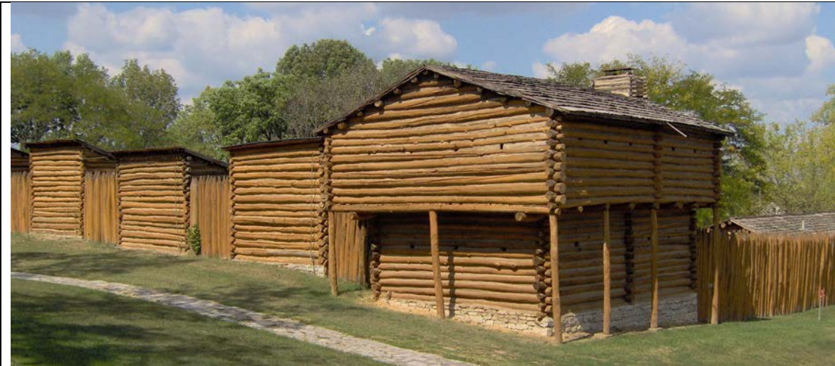
Fig. 2. Reconstruction of Fort Harrod located at Old Fort Harrod State Park in Harrodsburg, Kentucky. Built in 1775, Fort Harrod was the first permanent American settlement in Kentucky. Note the arrangement of cabins along the left wall with roofs sloping inward and the extension of the second floor of the blockhouse beyond the stockade wall. Photo credit: Wikimedia Commons [6].
